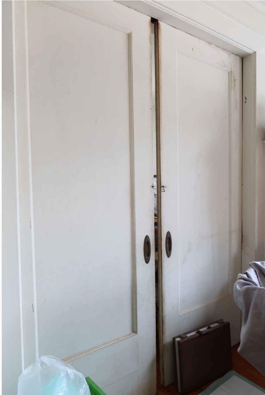
View of the pocket doors to the study from the southeast
