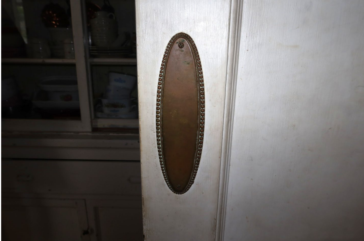
View of the dining room's swinging door's push plate from the south
