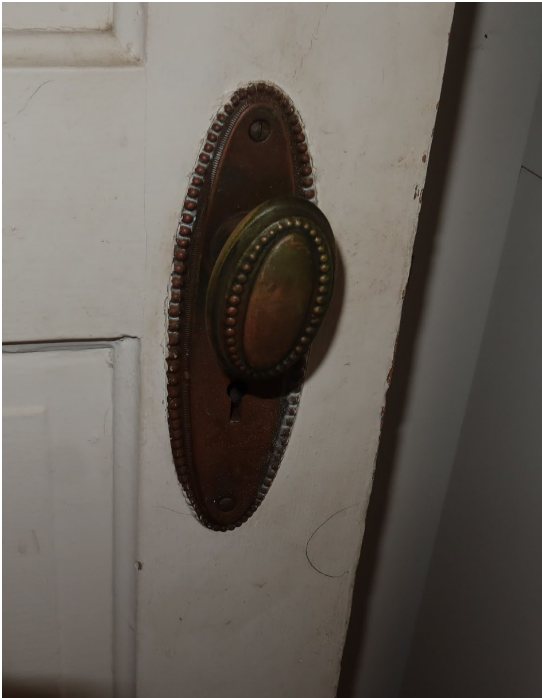
View of typical second floor doorknob from the west
