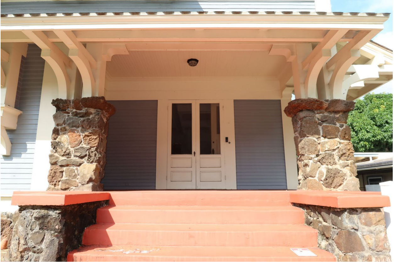
View of the entry porch from the east
