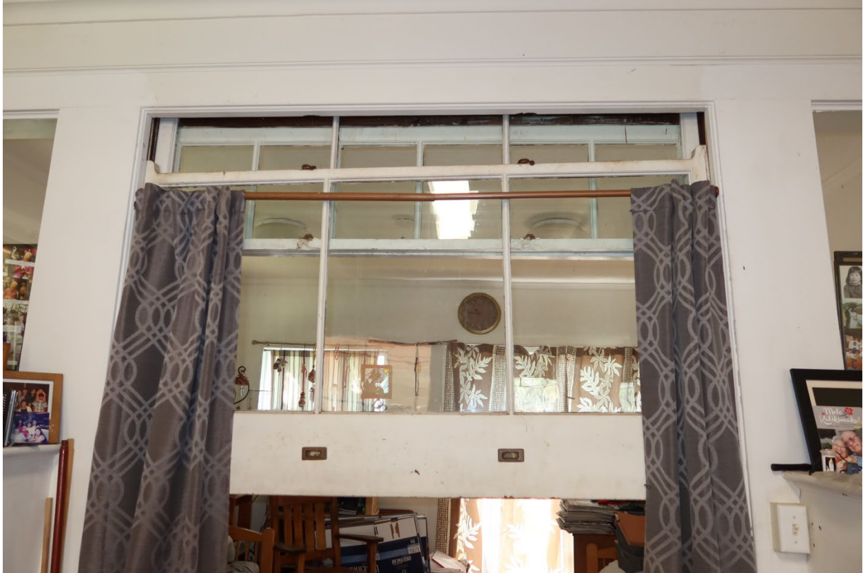
View of the dining room's vertical pocket window/door from the north
