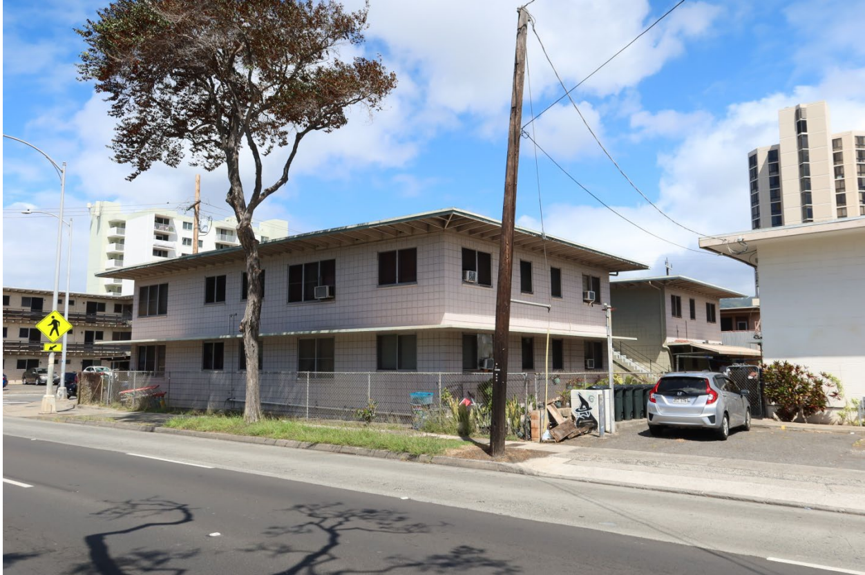
View of the six unit, makai apartment from Kapiolani Boulevard from the southeast
