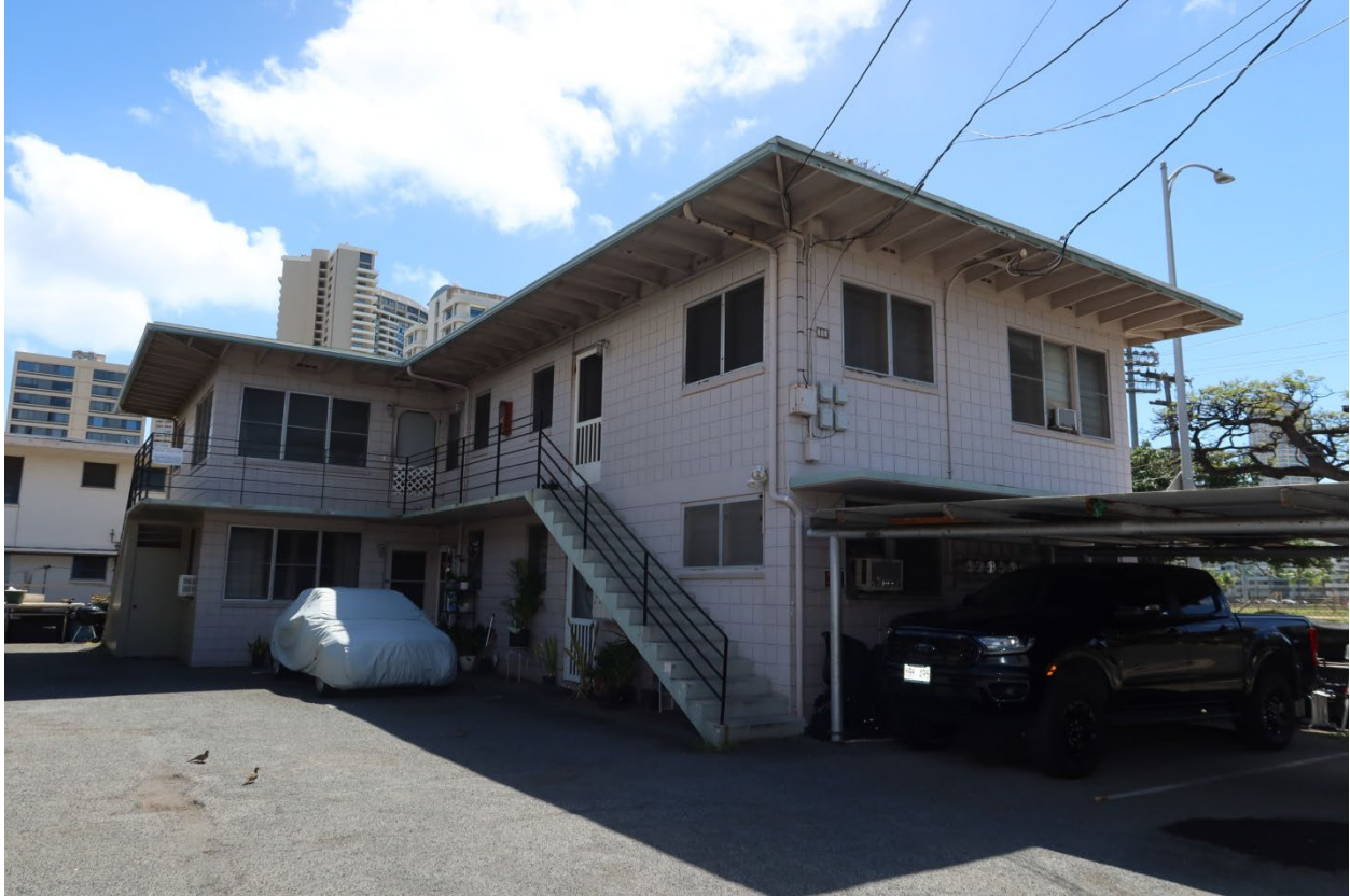
View of the front and side of the six unit, makai apartment from the northwest
