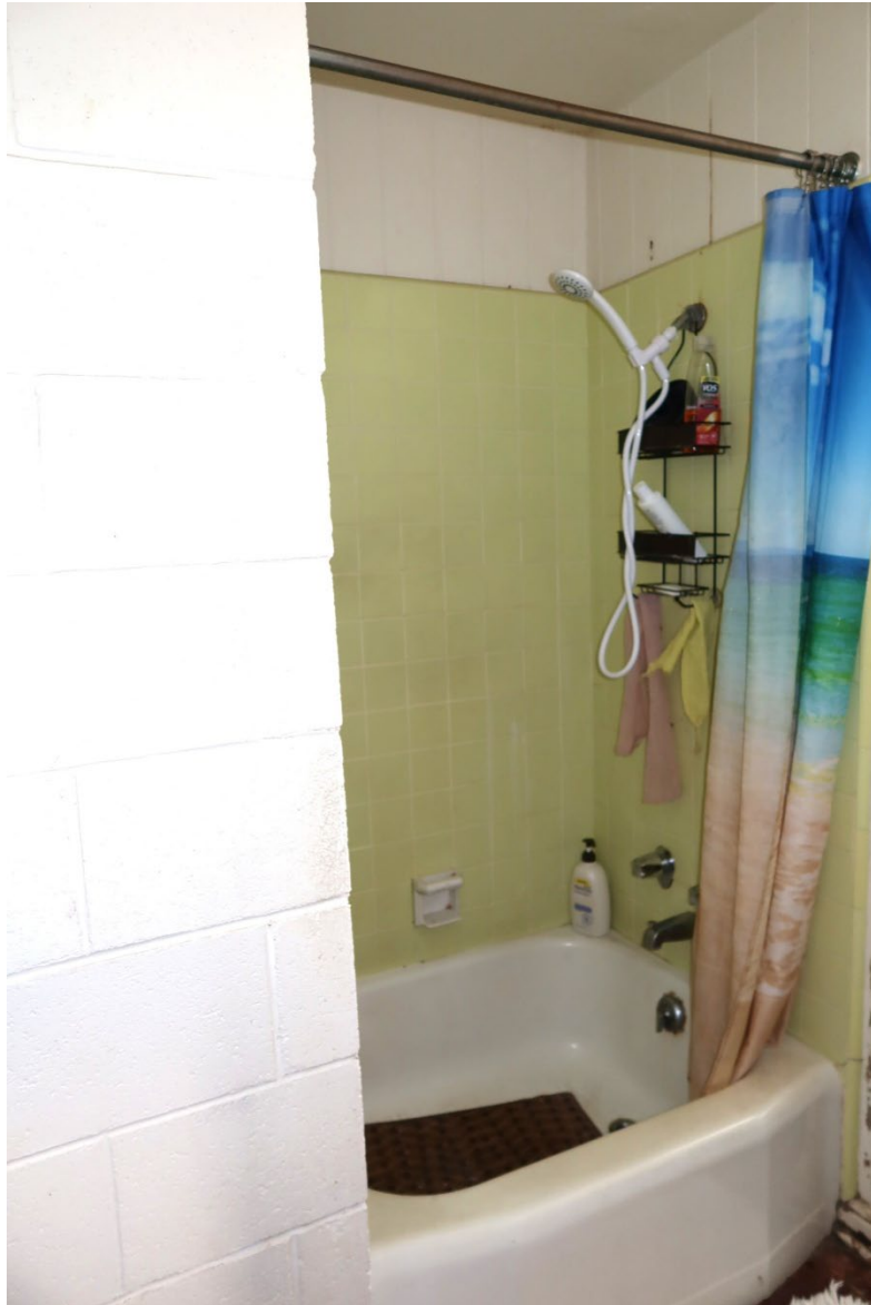
View of the shower from the northwest
