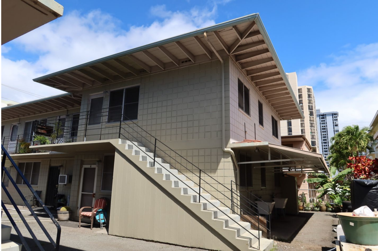
View of the east end of the eight unit, mauka side apartment from the south
