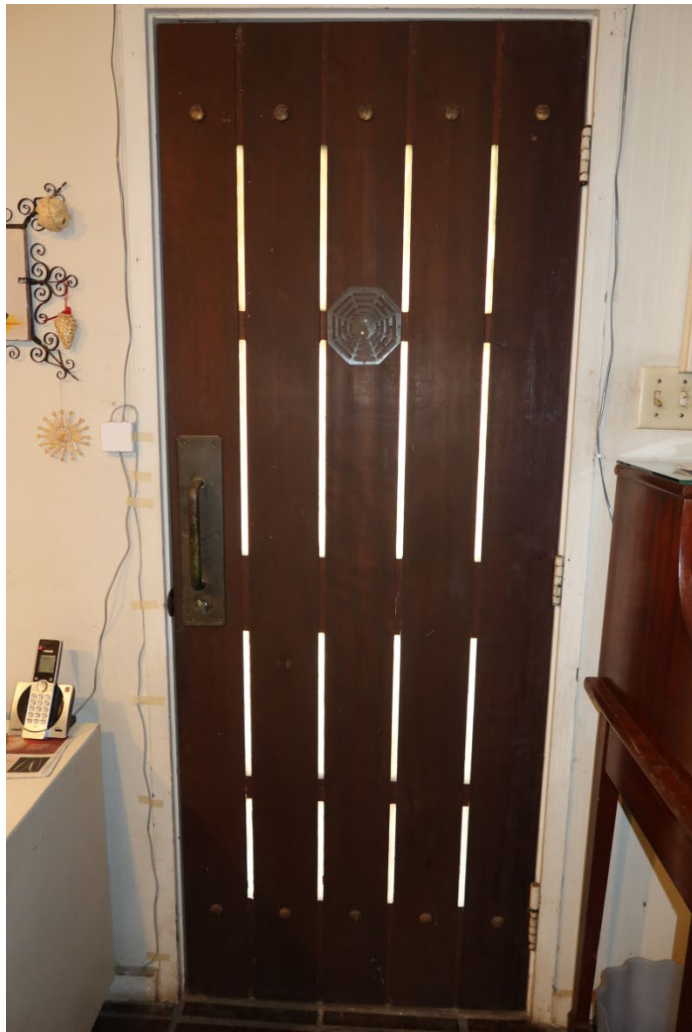
View of kitchen door to courtyard with Lucite inlays from the east
