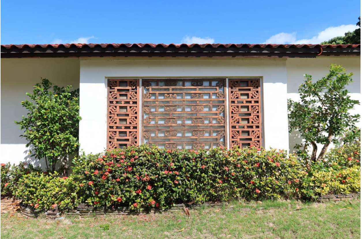
View of typical Chinese wood screen in front wall from the south
