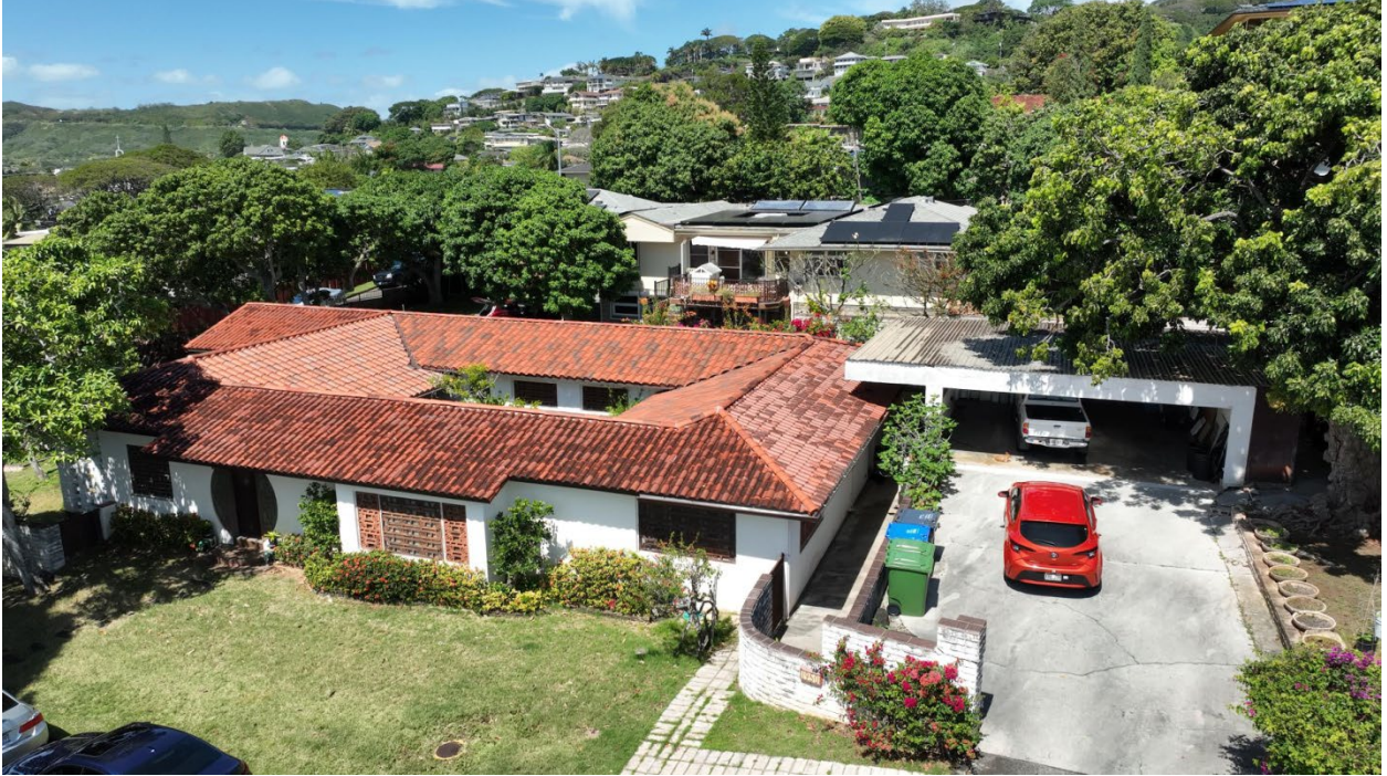
Drone view of the house from the southeast
