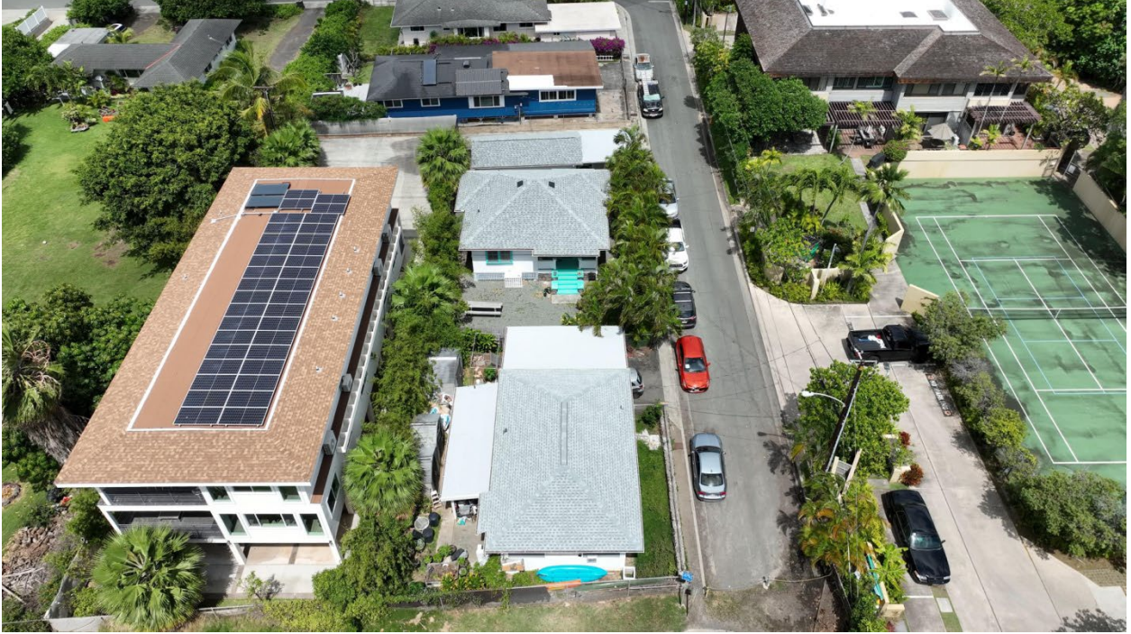
Drone view of the property from the south
