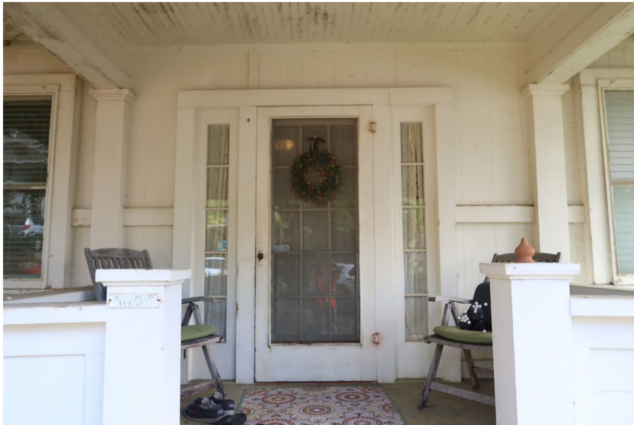
View of the entry from the west
