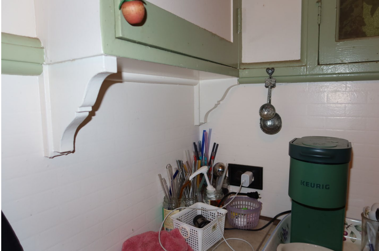
View of the butler pantry's bracketed cabinets and lincrusta wainscot from the east
