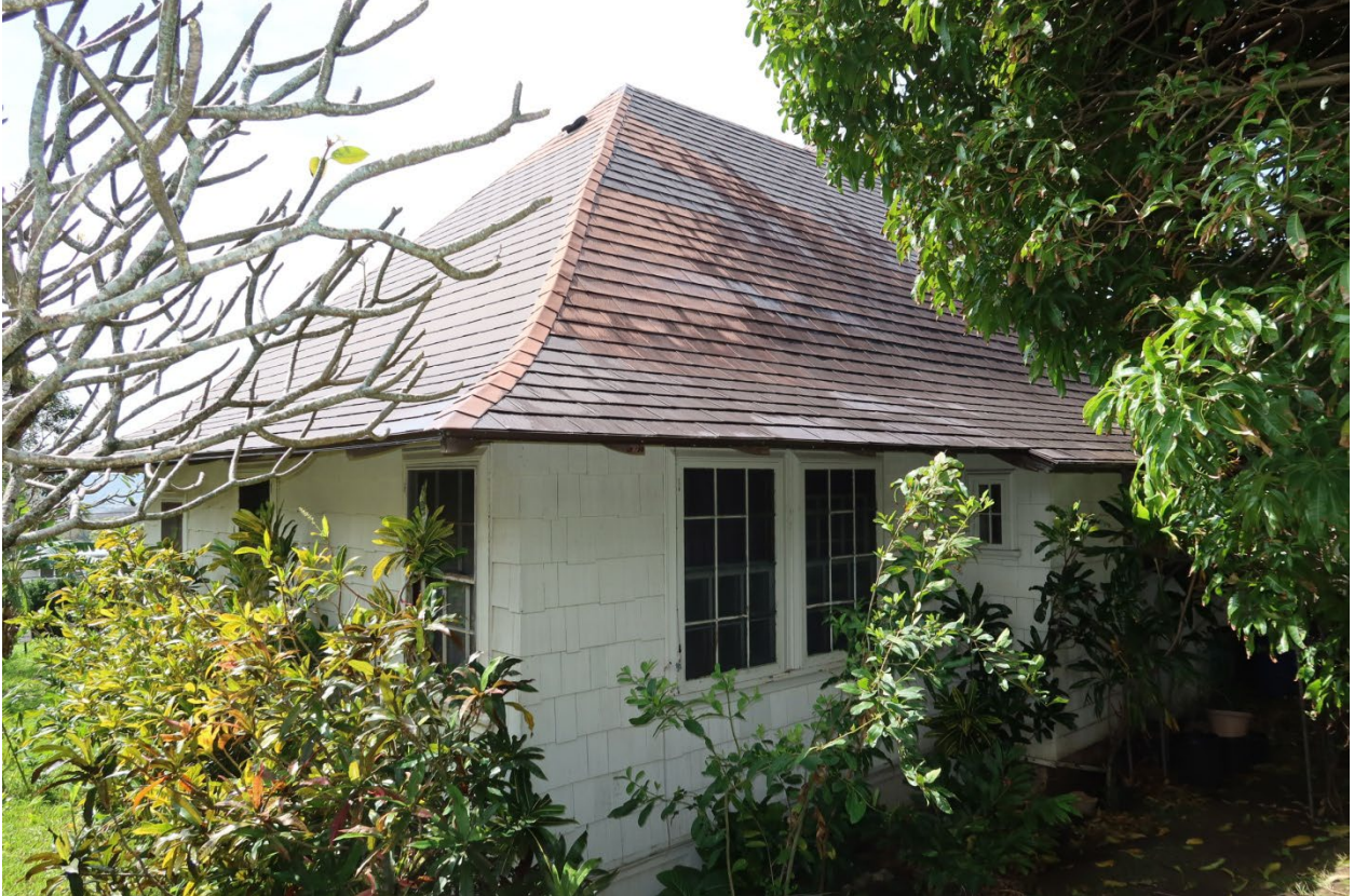
View of the east side and rear from the northeast
