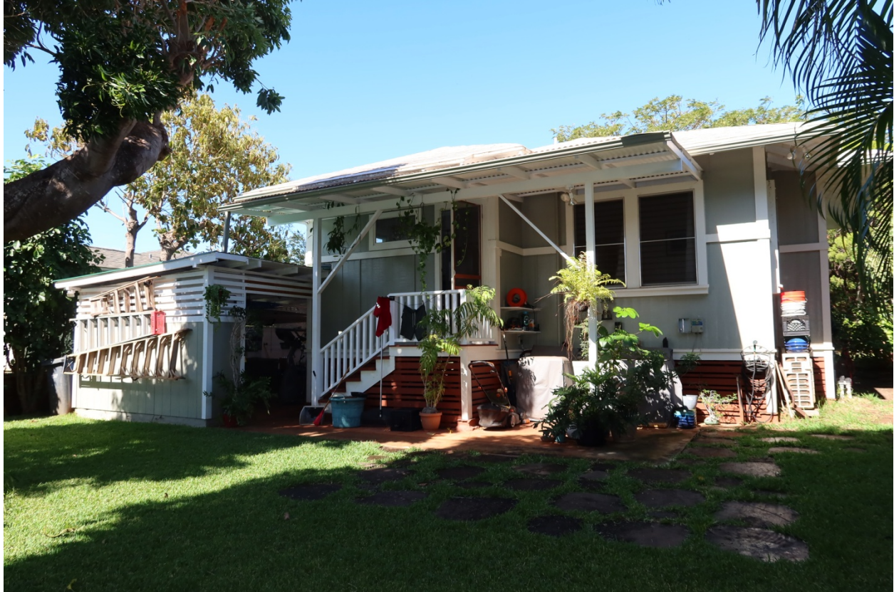
View of the rear of the house from the southeast
