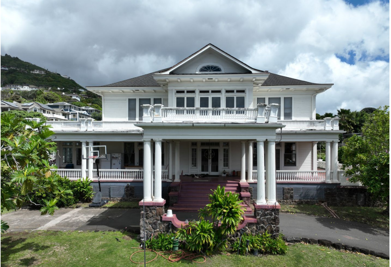
Drone view of the front of the house from the west
