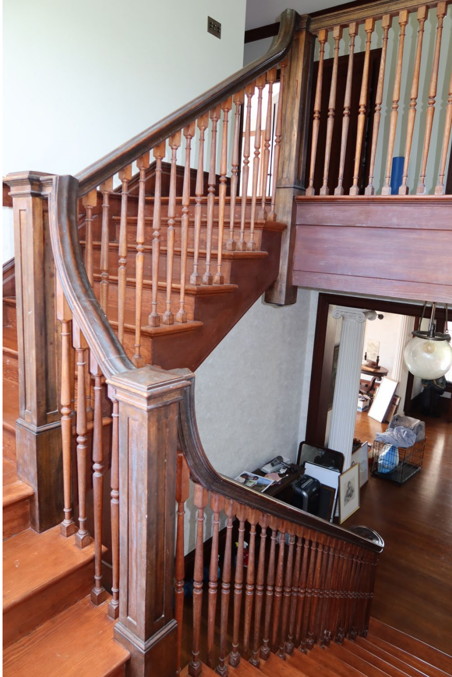
View of the stair from first landing from the northeast
