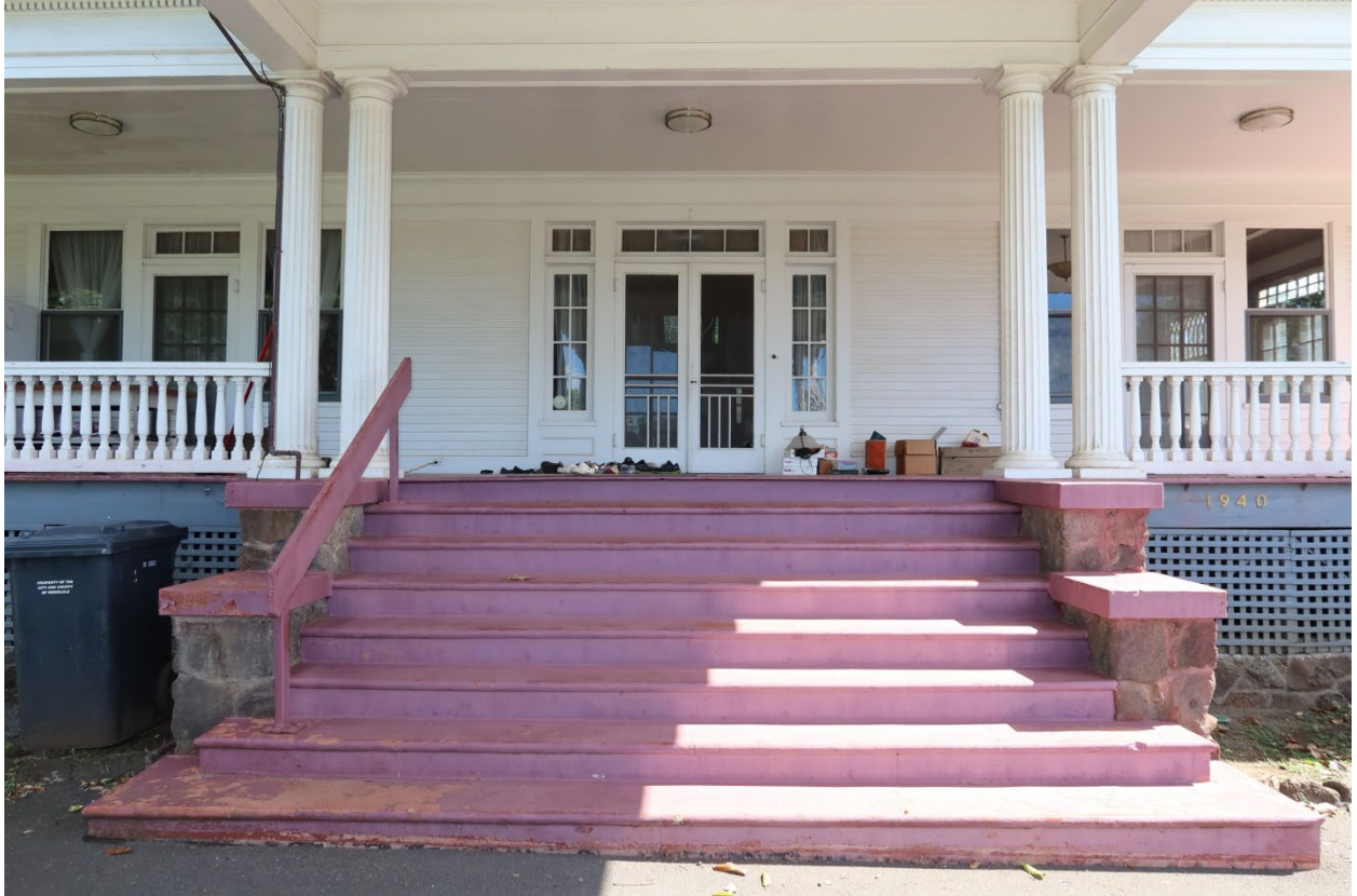
View of the entry from the west
