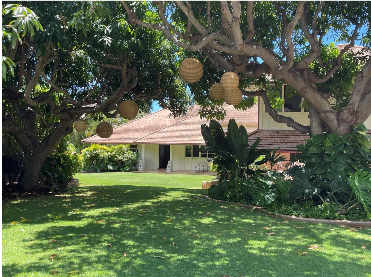
Photo 2 of 18 HI_Honolulu County_Cloward Residence_002. View to Main Entry, North (front) Façade. View to South.
