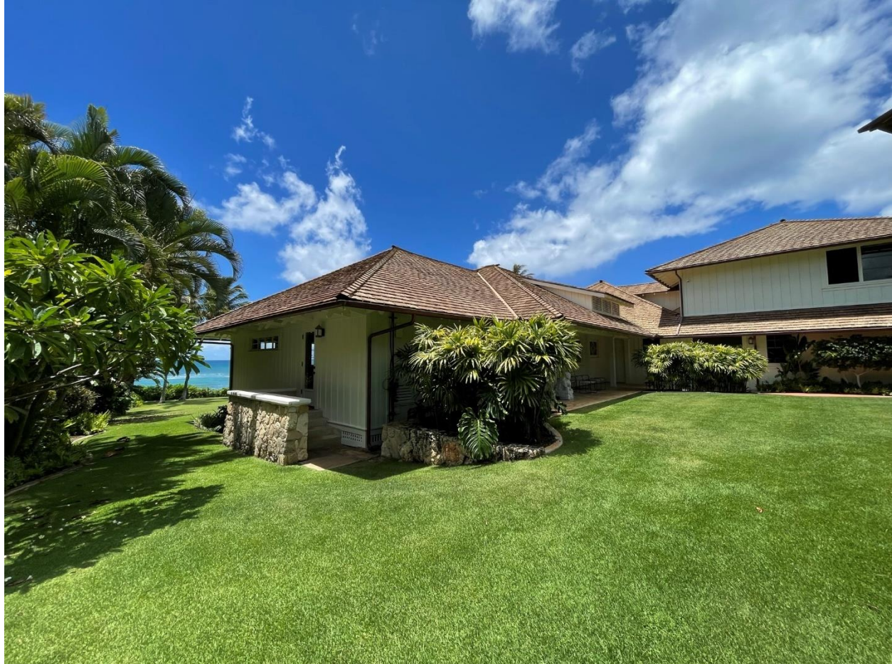
Photo 7 of 18 HI_Honolulu County_Cloward Residence_007. East Facade. View to Southwest.
