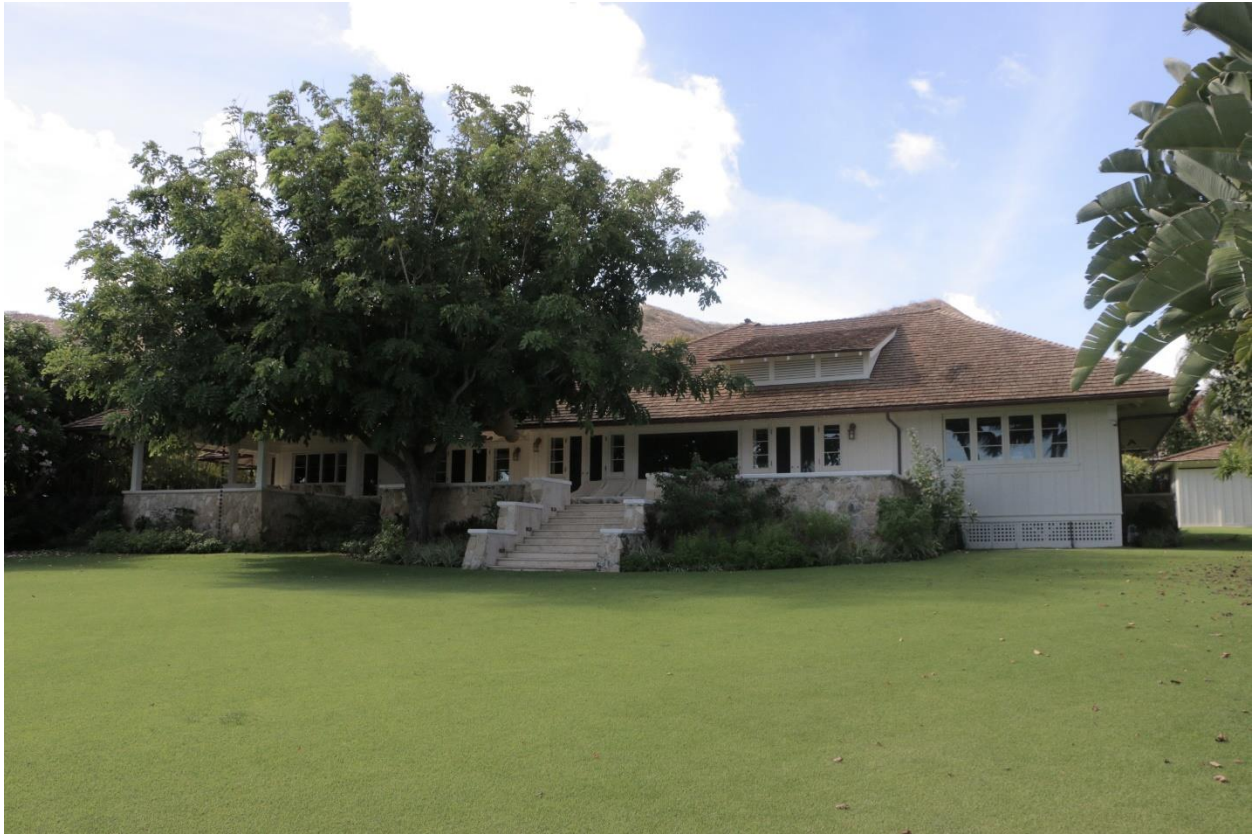
Photo 4 of 18 HI_Honolulu County_Cloward Residence_004. South (rear, beachside) Façade. View to Northwest.
