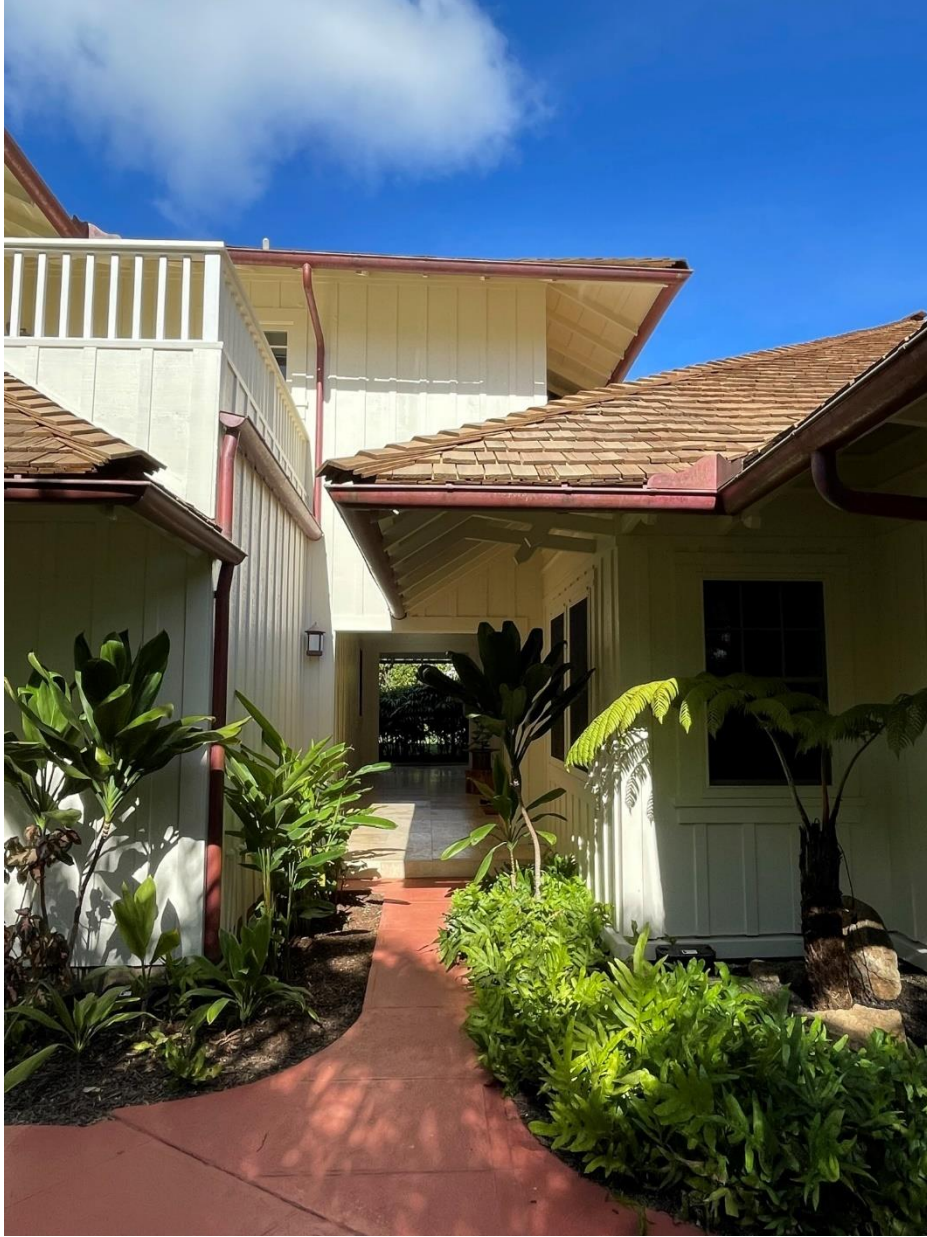
Photo 5 of 18 HI_Honolulu County_Cloward Residence_005. West Façade at Breezeway. View to East.
