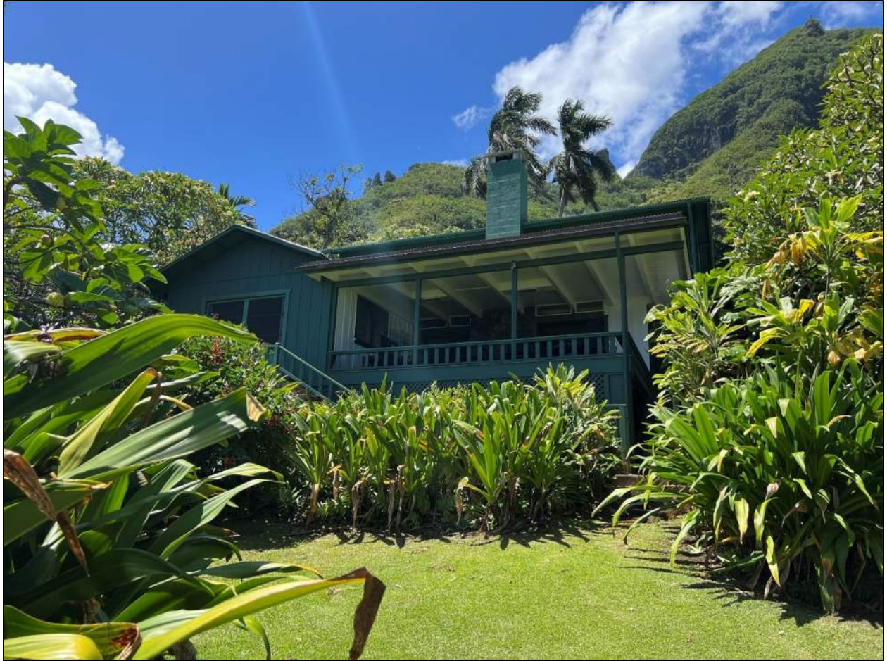
PHOTO 1 Of 18. Main House North Façade. View to South.
