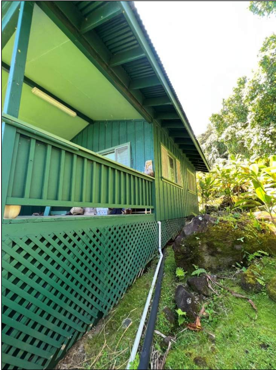
PHOTO 13 Of 18. House 3 West Façade. View to Southeast.
