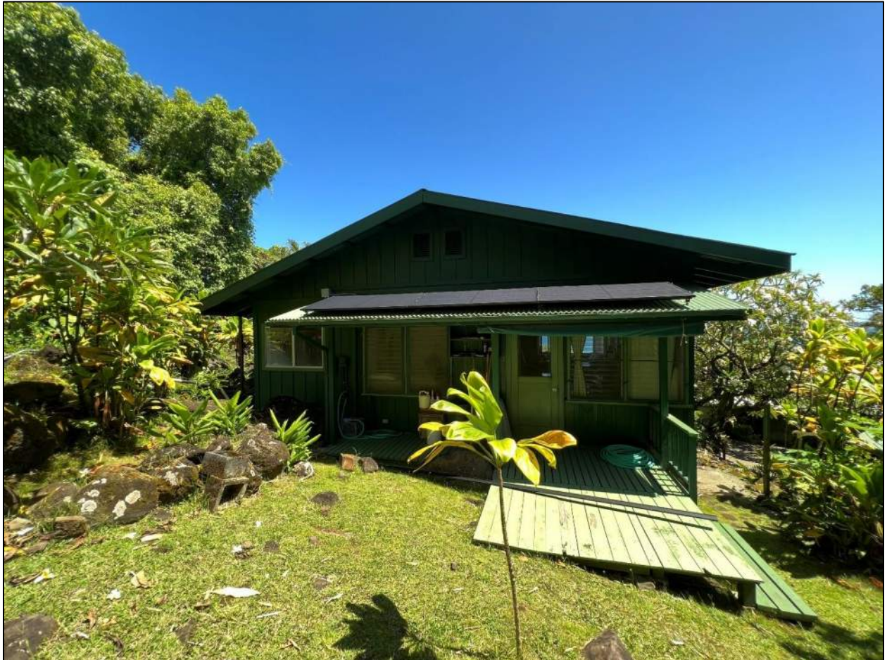
PHOTO 12 Of 18. House 3 South Façade. View to North.
