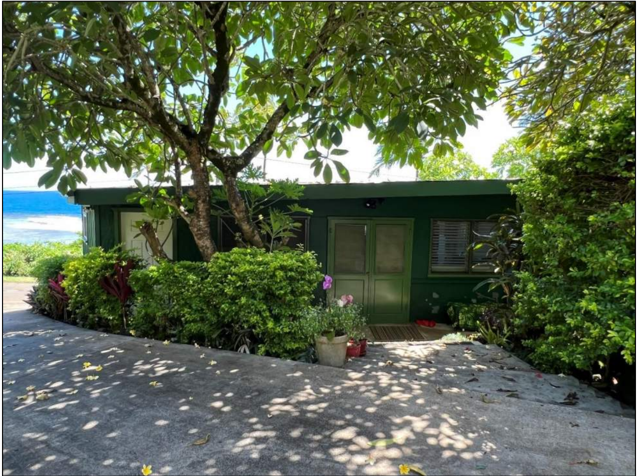
PHOTO 9 Of 18. House 2 South Façade. View to North.
