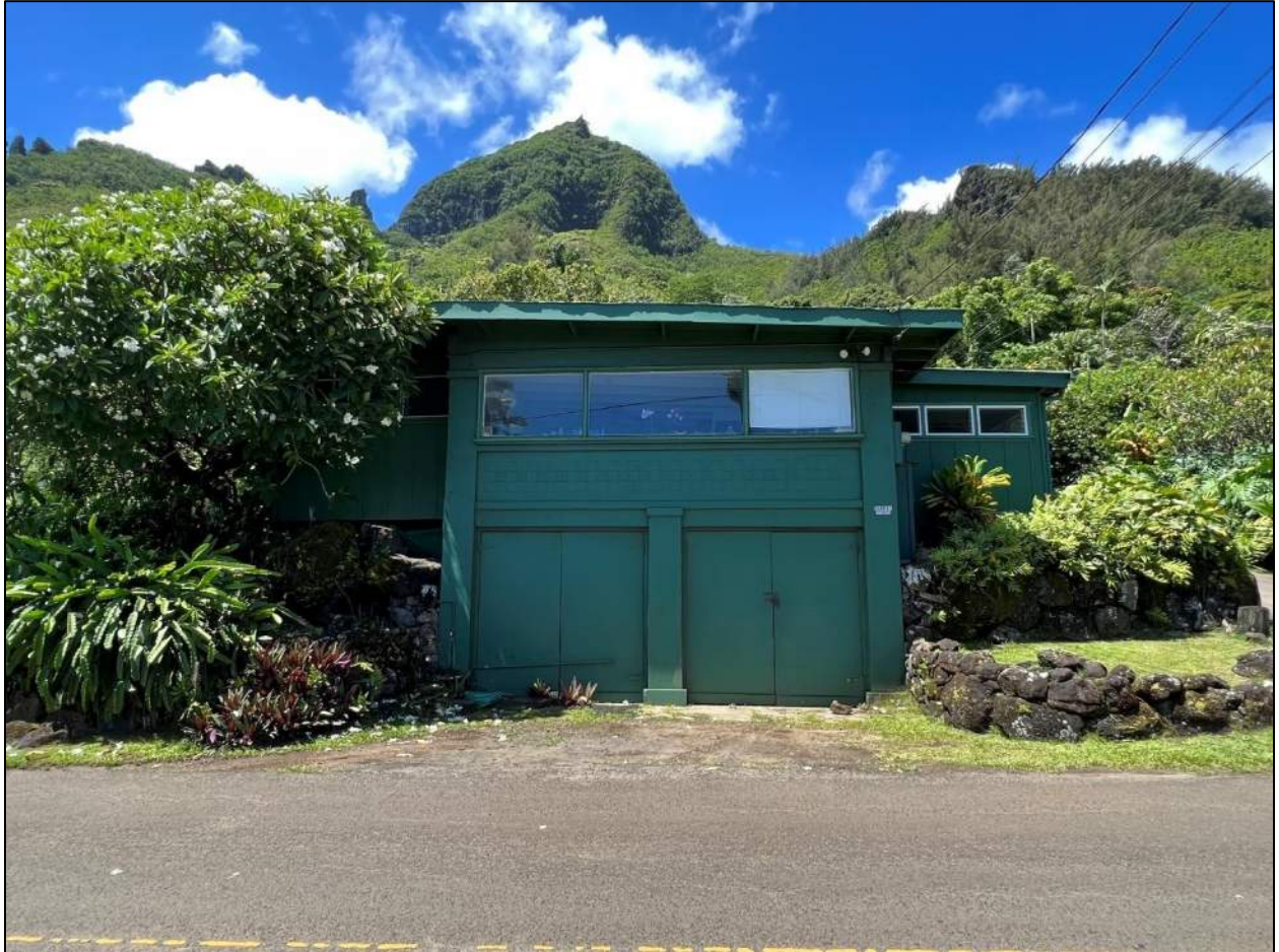
PHOTO 8 Of 18. Old Garage and House 2 North Façade. View to South.
