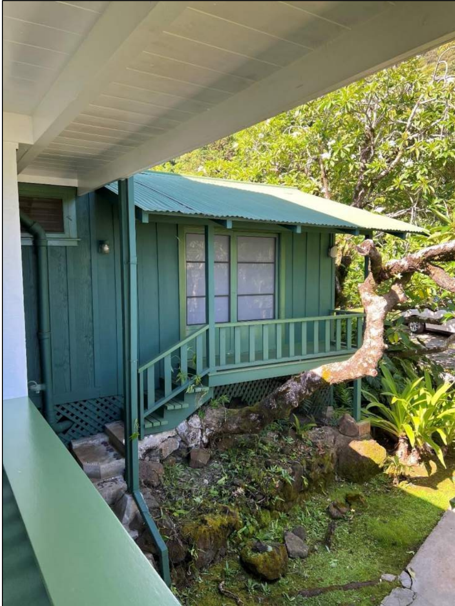
PHOTO 2 Of 18. Main House North Façade Guest Bedroom Wing. View to Southwest.
