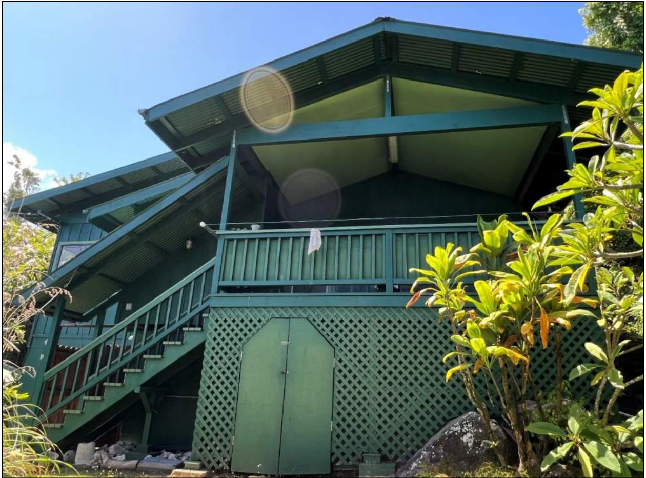
PHOTO 11 Of 18. House 3 North Façade. View to South.
