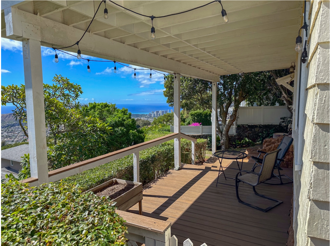
Photo 10 Daylight basement lanai on the makai (south) side of the Bowers' House looking southwest.
