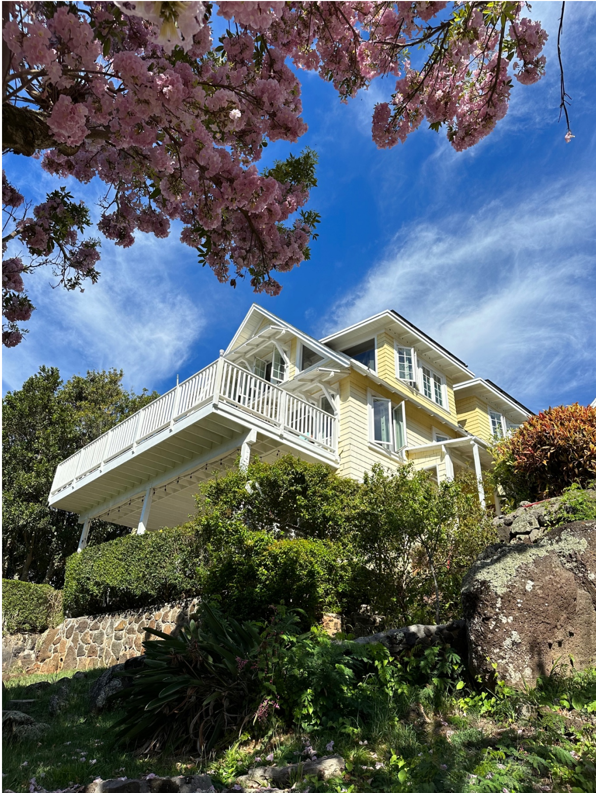
Photo 8 Bowers' House taken from the downhill side looking up to the northwest, with view of the deck/lanai on the south side of the house.
