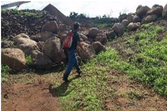
Wes Nohara, West Maui SWCD Associate Director conducting annual inspection of the Lahaina Temporary Flood Control Project. Boulders and trash were found within the trough, posing potential disaster in the event of a major flood.
