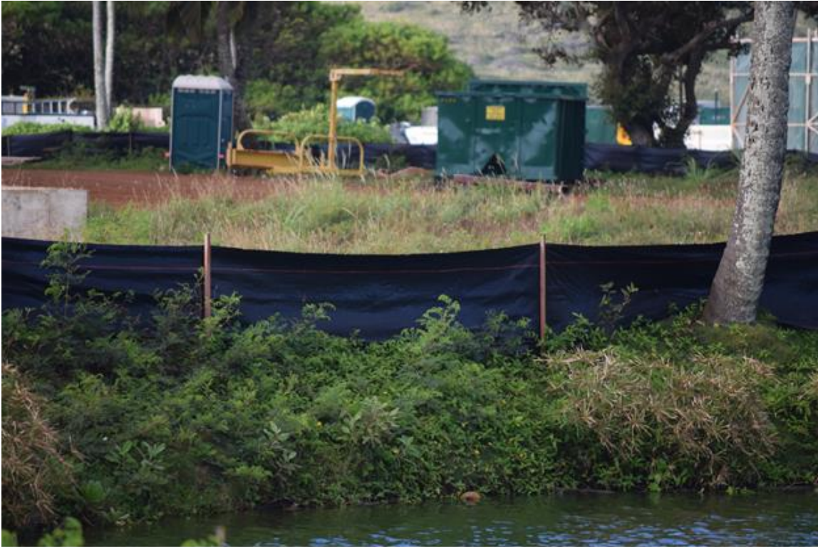
Image 6. Close-up of silt fencing
