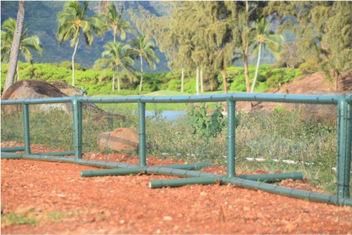
Image 5. Silt fencing inside the construction area
