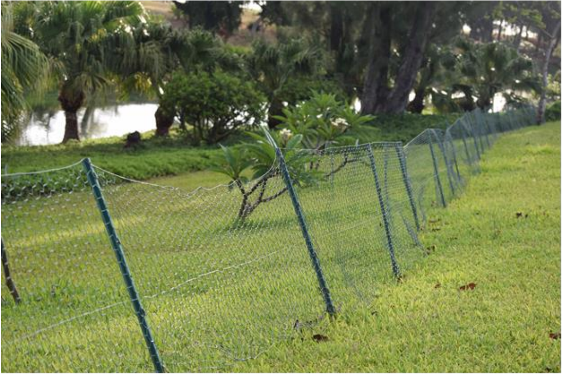
Figure 3. Mobile fencing section between pumping station and construction gate
