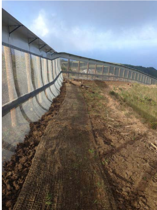
Figure 3. Jute matting around Enclosure B.
