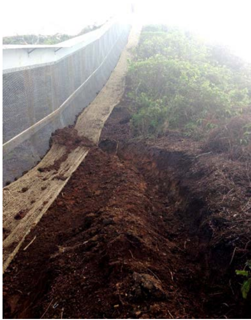
Figure 5. Recently completed water diversion and jute matting on the west facing slope of Enclosure B.
