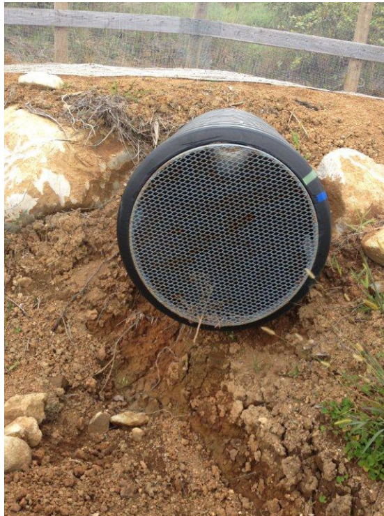
Figure 11. A screened culvert outlet before the rock apron is applied.
