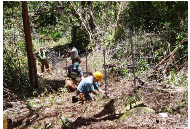
Ungulate fencing installation
