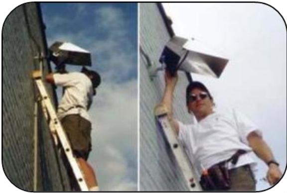
Figure 1: Installation of an appropriately sized floodlight shield. Source: www.darksky.org .
