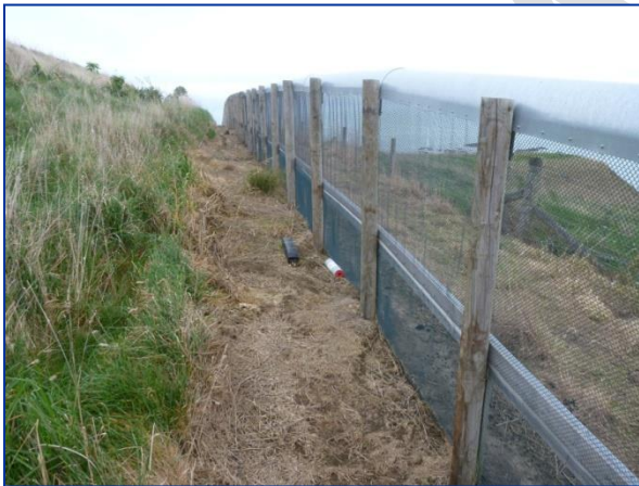
Figure 10.4. Similar predator-proof fence at Hutton's shearwater colony, Kaikoura, New Zealand. A Raine.
