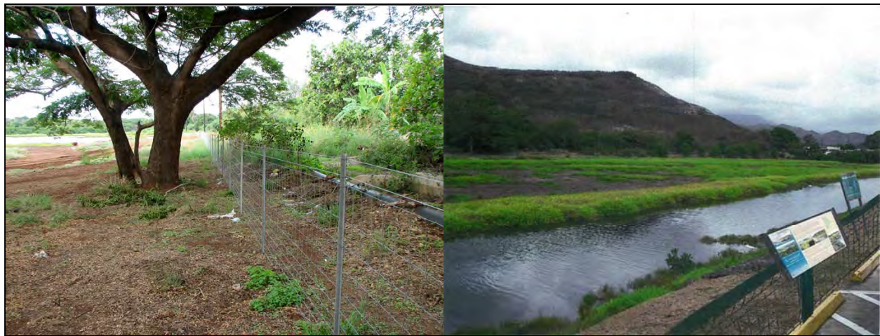
Exhibit 2.15 Typical Perimeter Wire Fencing and Fencing Option with Interpretive Signage
