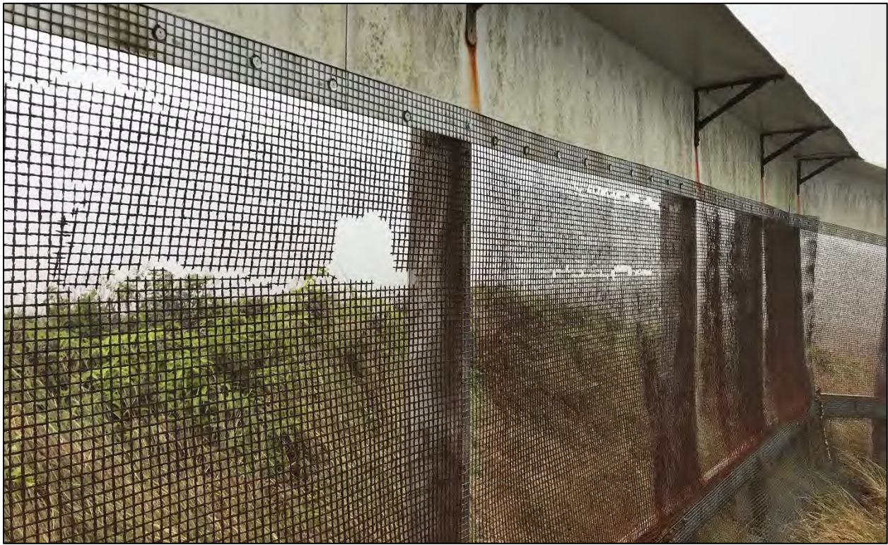
Figure 2. Fence Damage Caused by Excessive Rust Detected in August 2019
