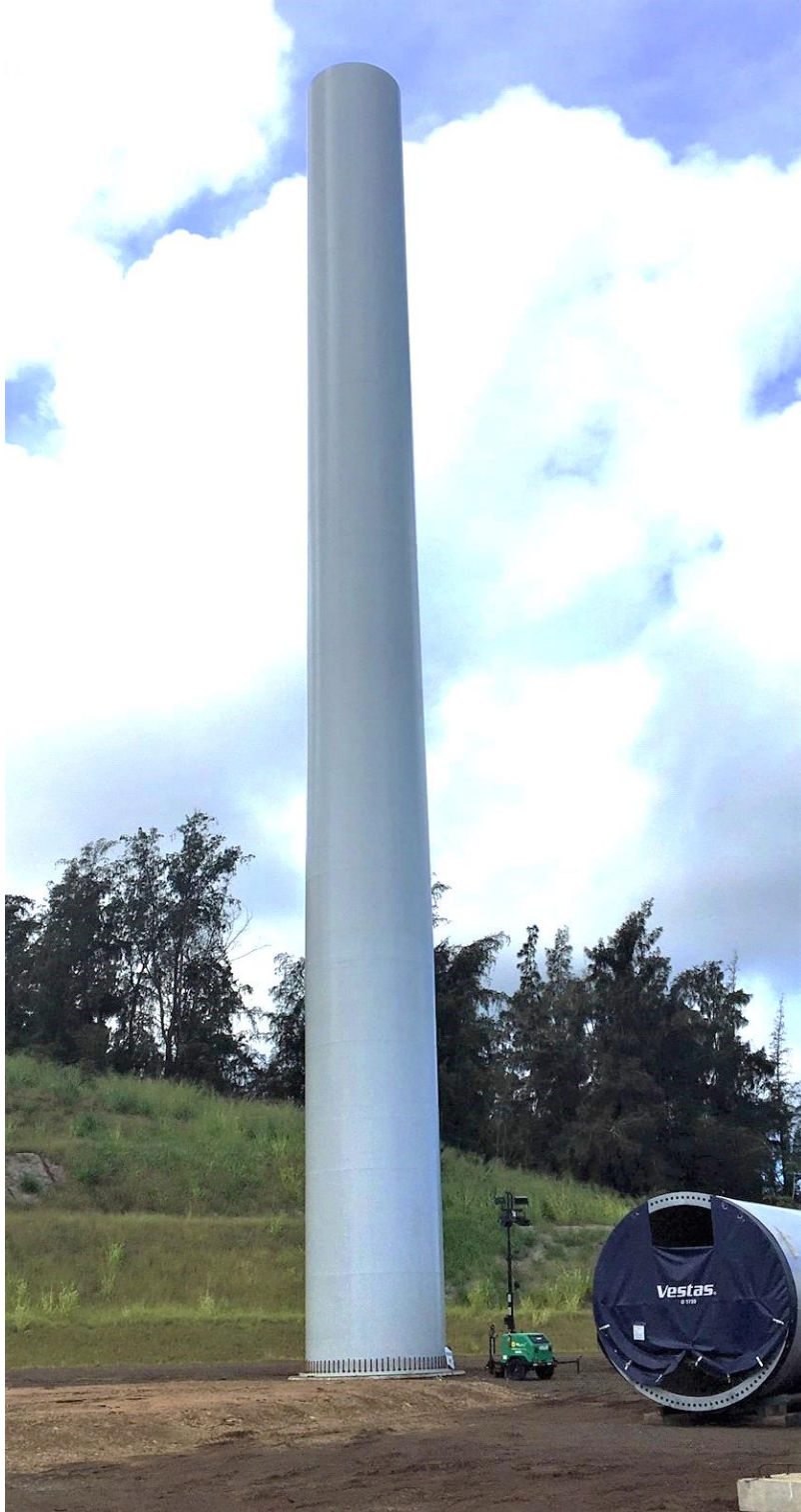
Figure 1. Security Light at Turbine 4
