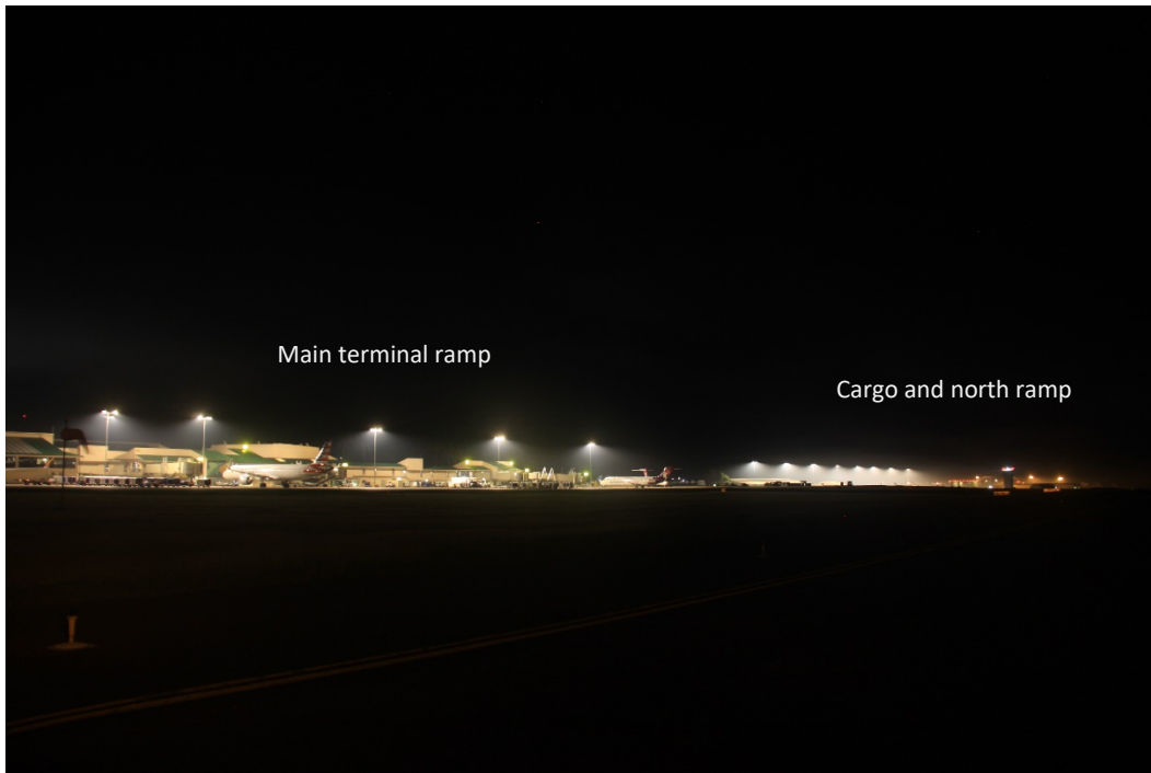
Photo 3 (top) and 4 (bottom). These images show the northern portion of the main terminal ramp and adjacent cargo ramp lighting at Lihue Airport in operational setting. High mast full cut off fixtures facilitate the direction of light at a downward angle.
