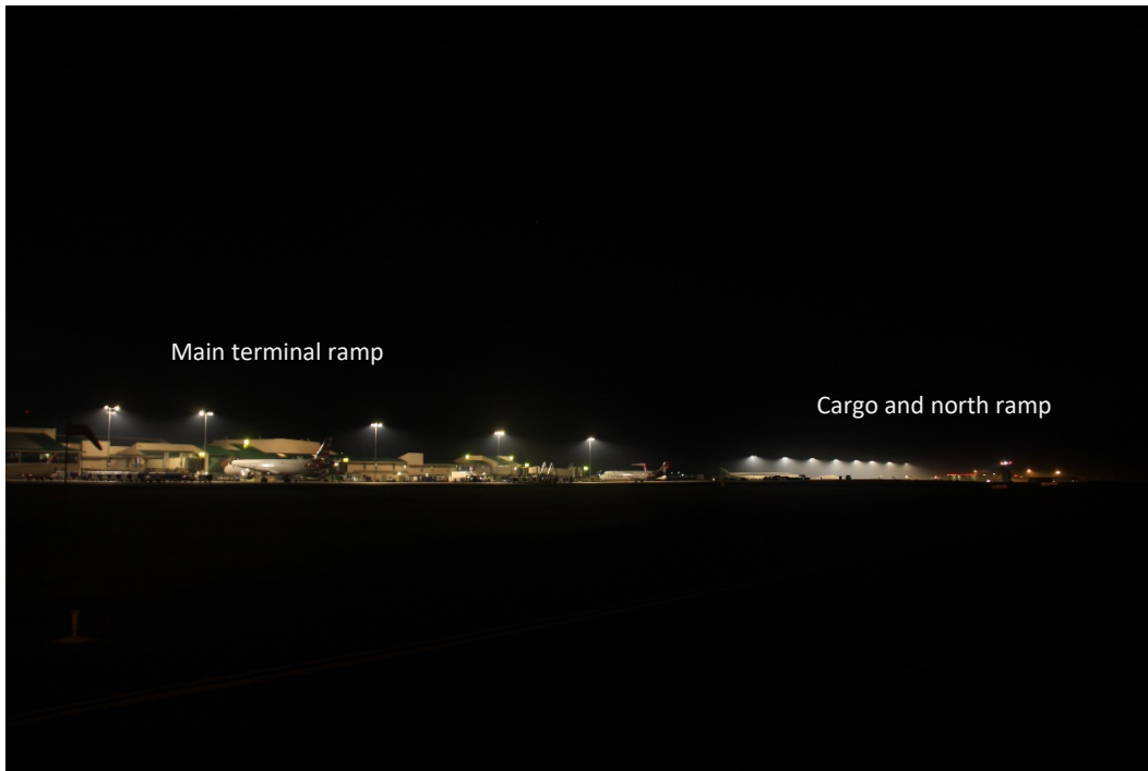
Photo 3 (top) and 4 (bottom). These images show the northern portion of the main terminal ramp and adjacent cargo ramp lighting at Lihue Airport in operational setting. High mast full cut off fixtures facilitate the direction of light at a downward angle.
