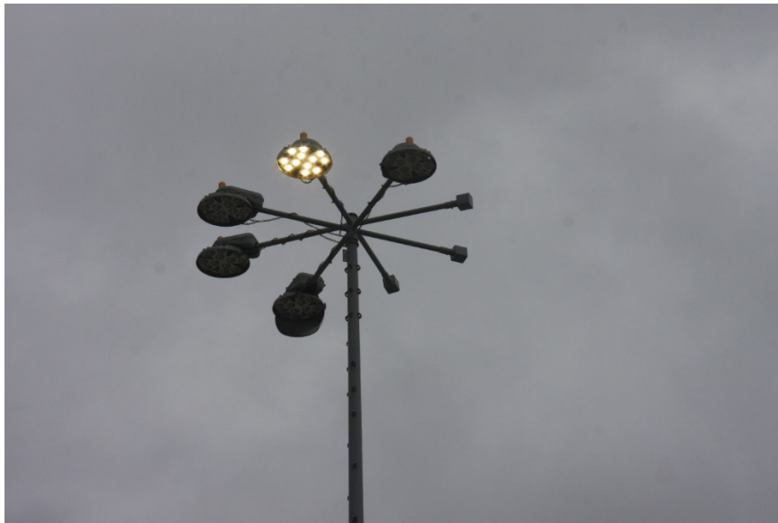
Photo 2. High mast light at Pier 1 (Matson yard) operating in a security setting – no operations, full minimization level.
