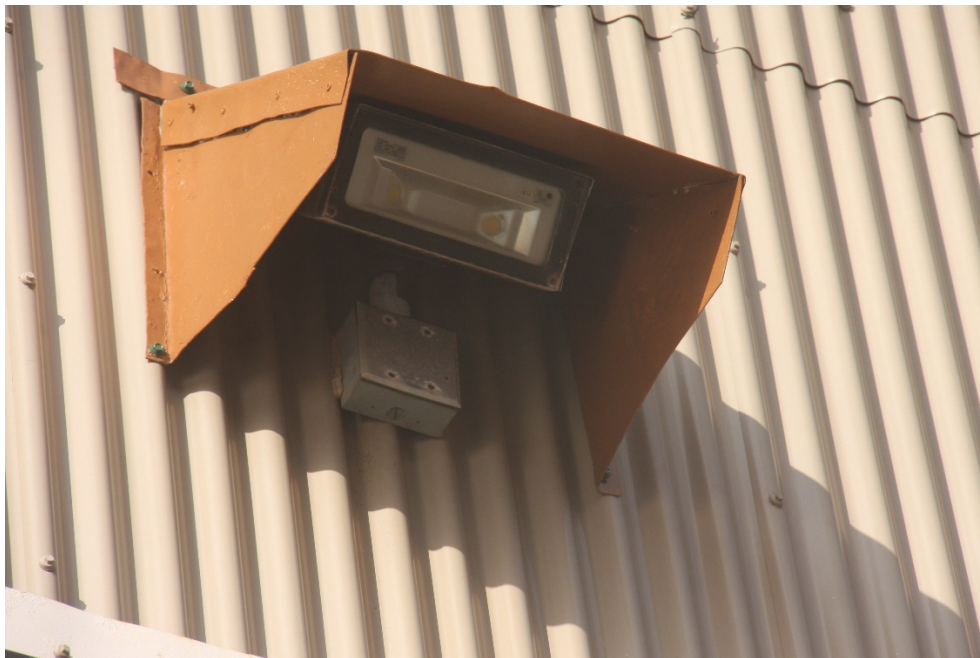
Photo 1 (above) presents a view along the south side of the main warehouse and pier at Port Allen Harbor with the newly installed siding and paint. Photo 2 (below) provides a view of the shielding that was installed on the main warehouse light in 2022.
