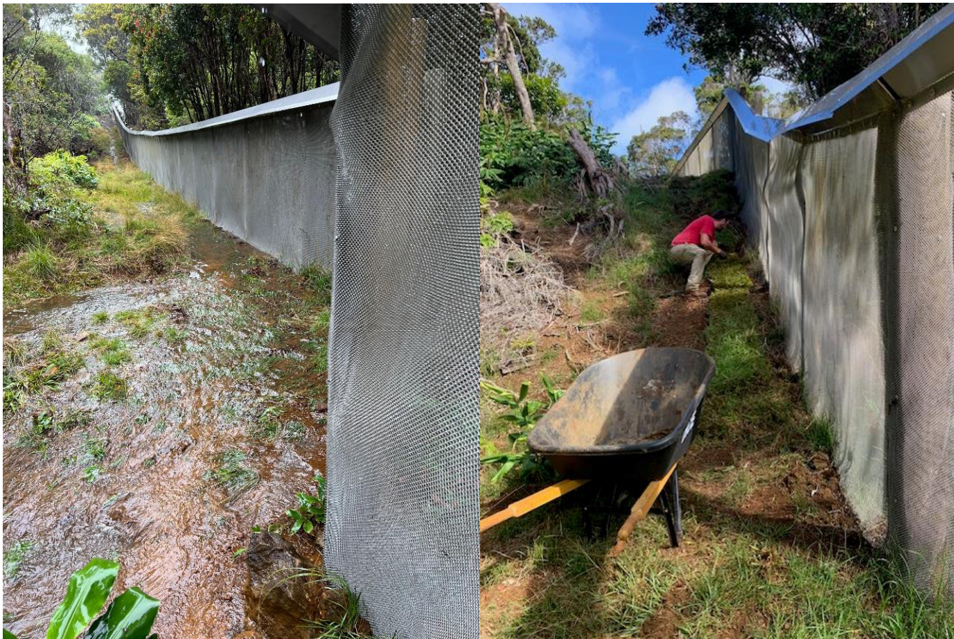
Figure 1: Images showing extensive flooding (left) followed by fence skirt re-attachment and sod placement (right)
