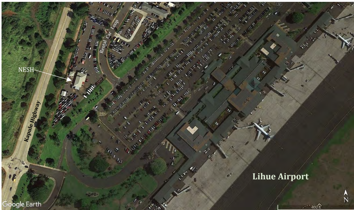
Wide view of the western end of Lihue Airport. The Newell's shearwater was discovered in one of the several rental car facilities that are adjacent to Kapule Highway
