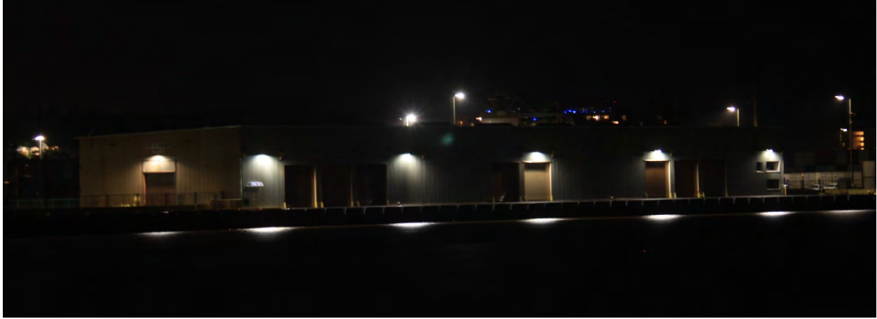
Photo 3. Wall-mounted lights illuminating bay doors and bulkhead along Pier 2.
