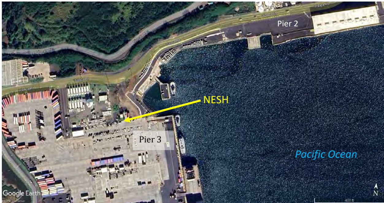
Overview of harbor facilities and infrastructure where the Newell's shearwater was discovered at Nawiliwili Harbor on October 9, 2023.
