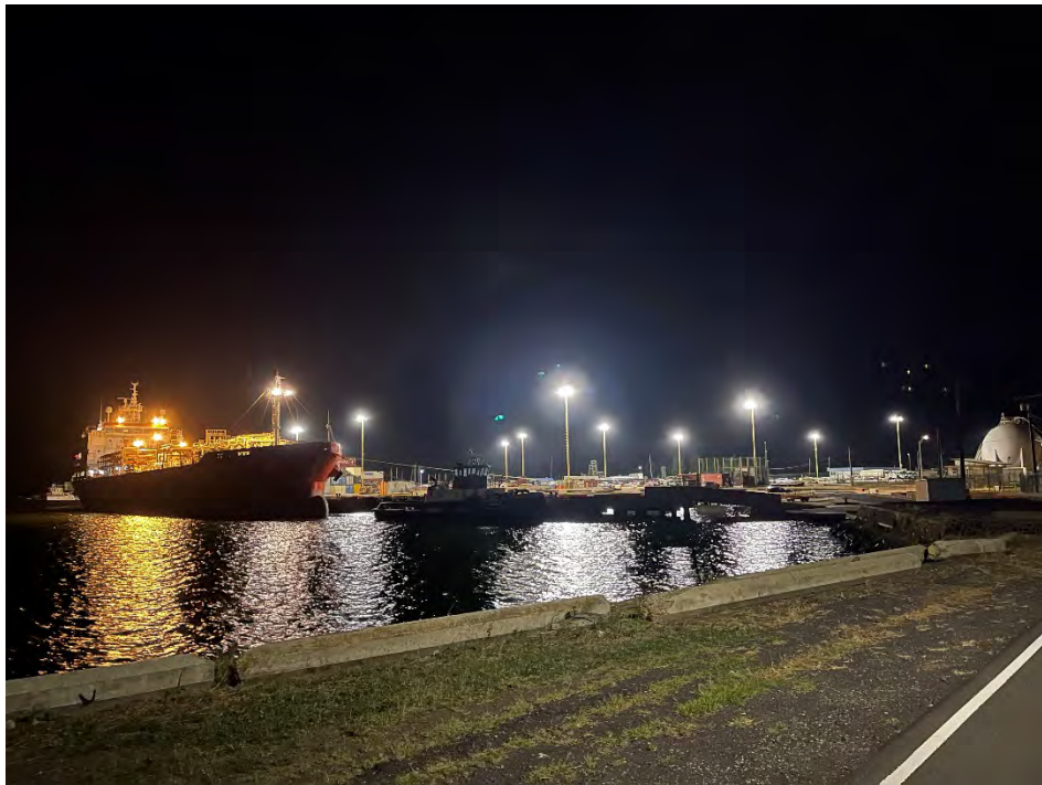
Photo 6. Lighting conditions at Pier 3 during bulk fuel operations.
