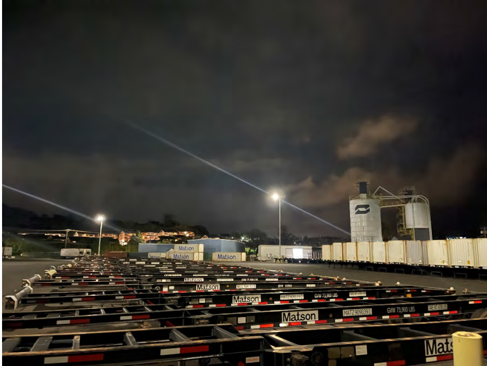
Photo 7. High mast lights in security setting at Pier 1.
