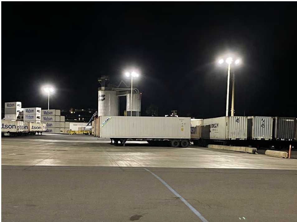
Photo 8. High mast lights in operational setting at Pier 1, Nawiliwili Harbor.
