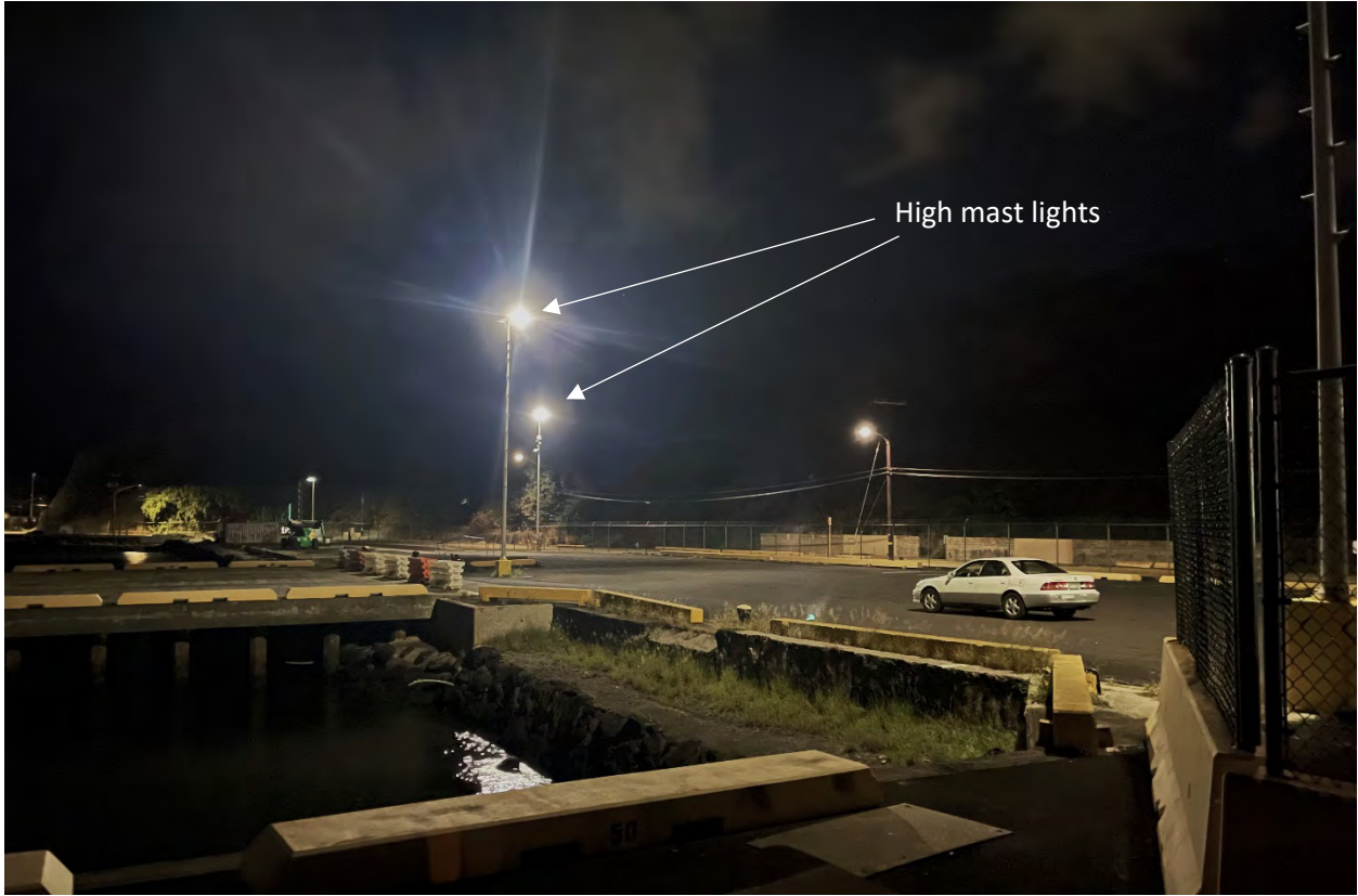
Photo 4. Two high mast lights between Piers 2 and 3 just to the southwest of the Pier 2 warehouse and cruise ship terminal.
