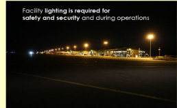
Facility lighting is required for safety and security and during operations.
