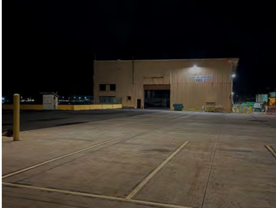
Photo 5. Wall mounted light on the side of the Pier 2 warehouse (east side facing Pier 1). This light typically remains on during both operational and security light level settings.
