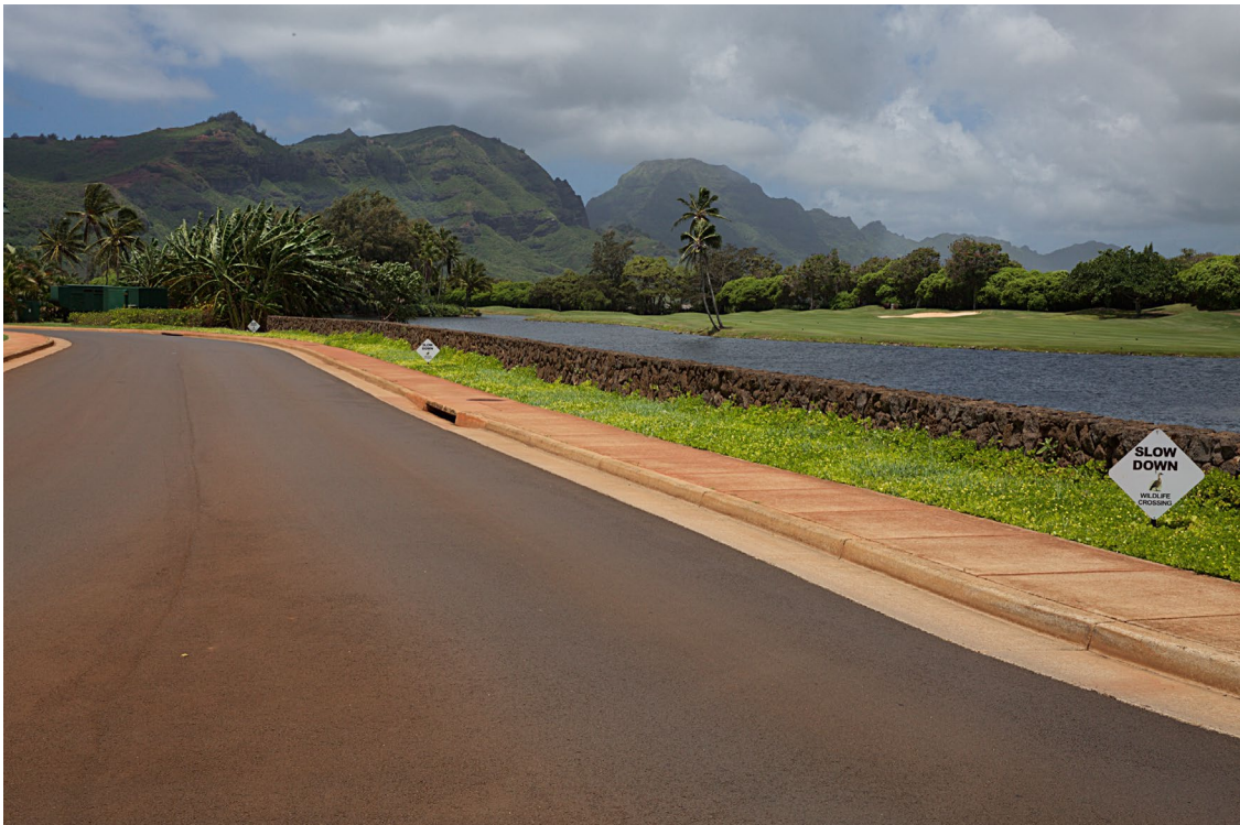
Figure 15 – Wildlife slow down warning signs placed every 45 feet along Holokāwelu Road.
