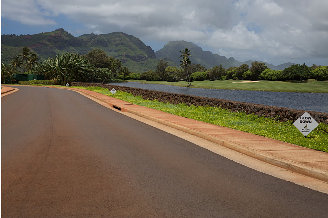
Figure 16 Wildlife slow down warning signs placed every 45 feet along Holokāwelu Road.
