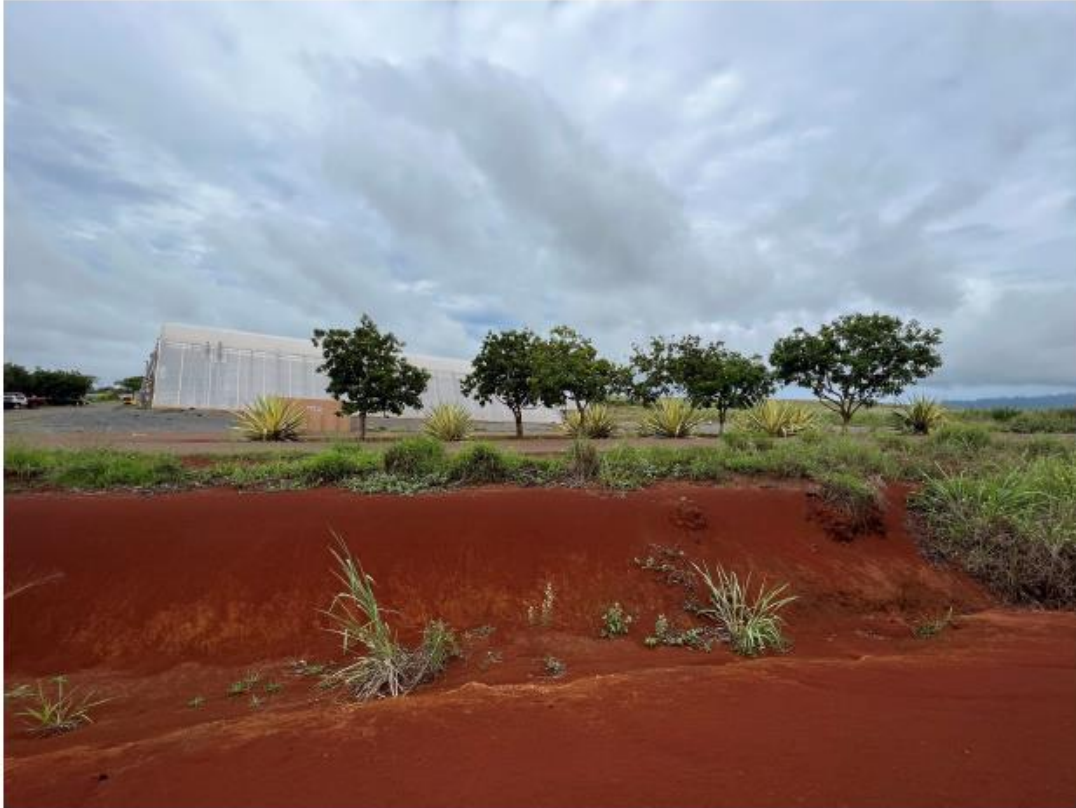
Drainage area at Sensei Farms hydroponic facility
