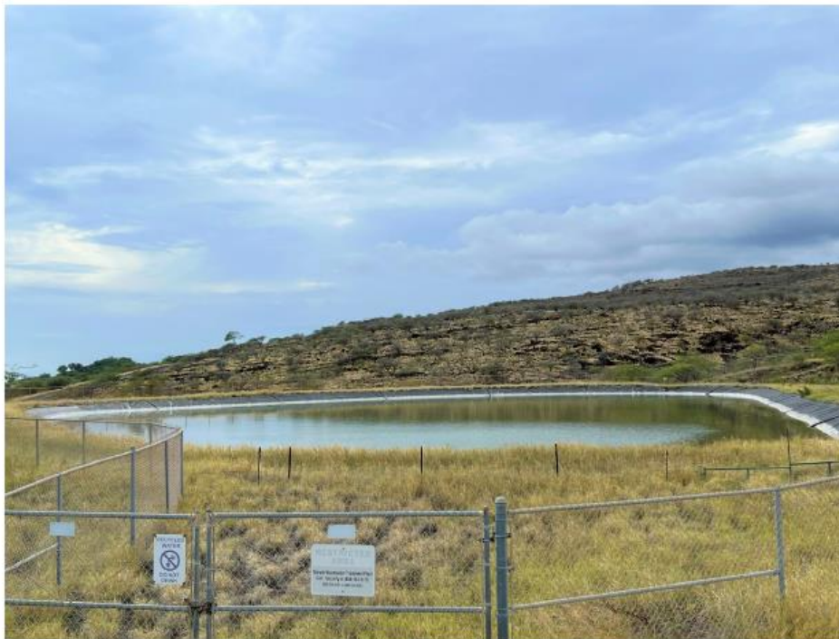
Open pond at the Mānele Wastewater Treatment Facility
