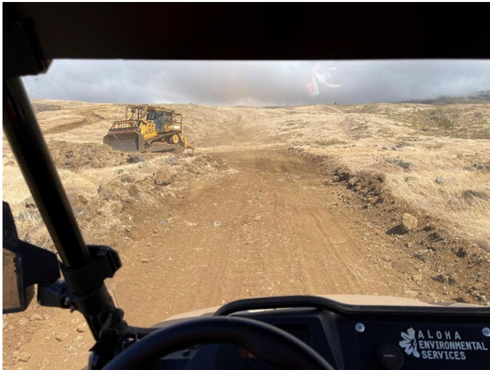
Photo 1. Bulldozer conducting access road maintenance in September 2023.
