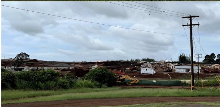
Hōkūau Residential Development under construction
