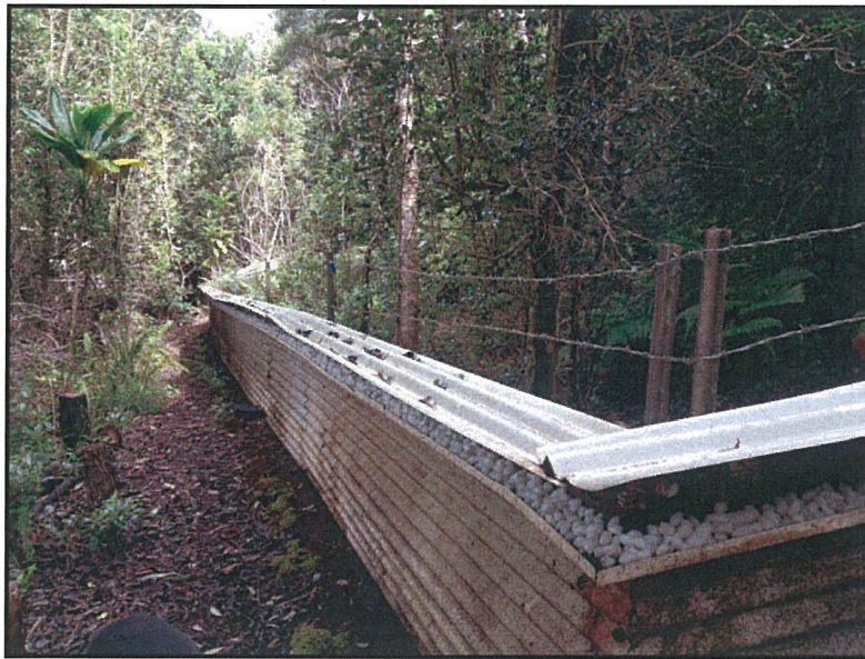
Exhibit 3. Current Pahole predator-proof enclosure structure. This structure was completed in 1998. Note rust and corrosion as a result of continual salt exposure.
