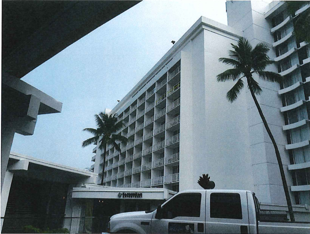
View of Mauna Kea Tower
