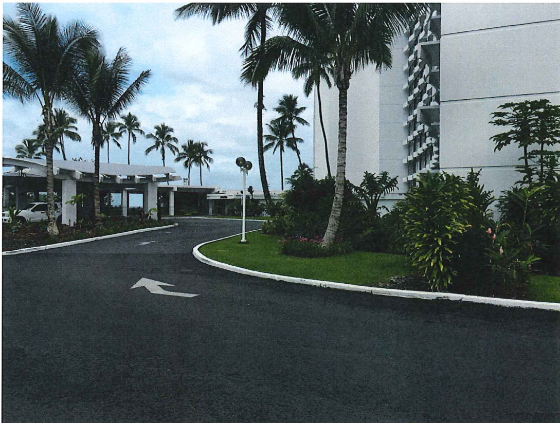
Entrance to Lobby Area
