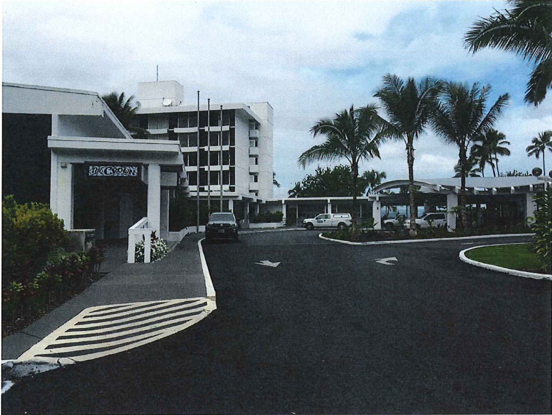
Entrance Showing Porte-Cochere
