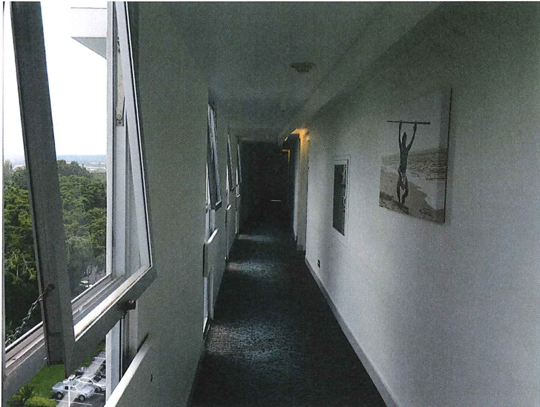
Newly Carpeted Hallway – Mauna Loa Tower
