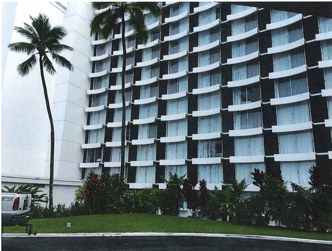
Newly Renovated Mauna Loa Tower
