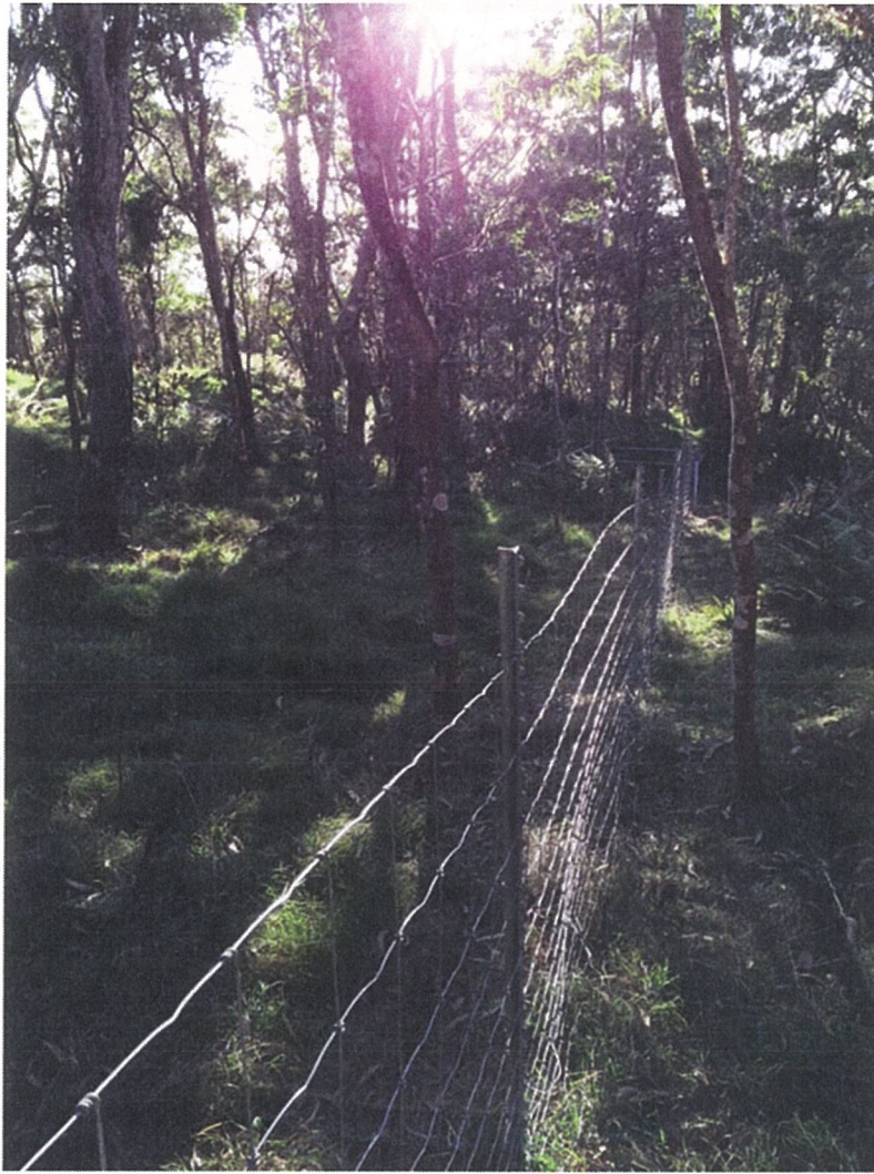
Figure 11 Four foot high hogwire fence with ground skirt for existing 0.8 acre enclosure illustrating the need to hand-cut fence lines in the dense forest. The proposed perimeter fence would be six feet tall.
