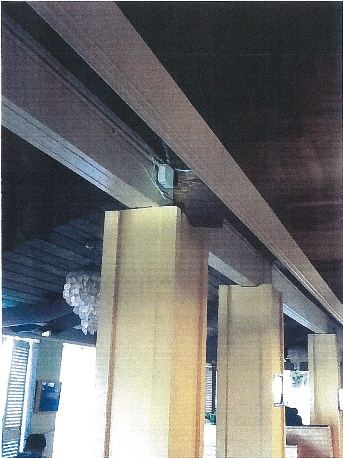
Rafter support evidencing termite damage and deterioration at load bearing [HCC5-48(2(F))]
