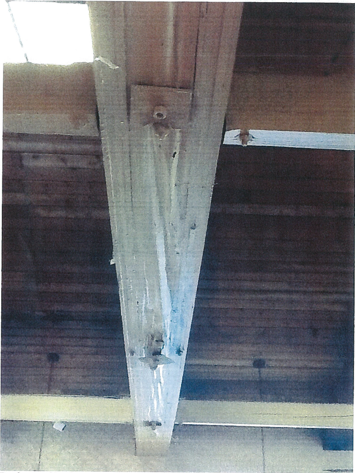
Roof truss evidencing termite damage and loosened hardware [HCC 5-48(2)(F)]
