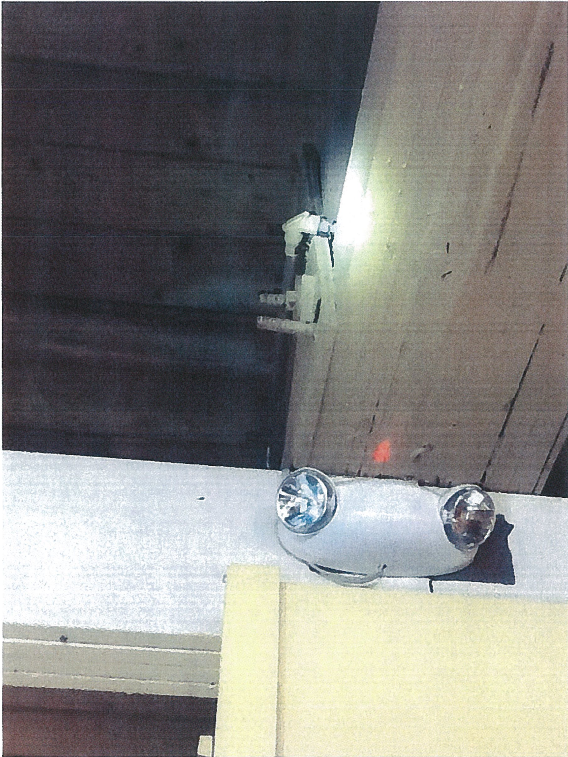
Roof truss connection plates missing (bolt) hardware [HCC 5-48(2)(F)]
