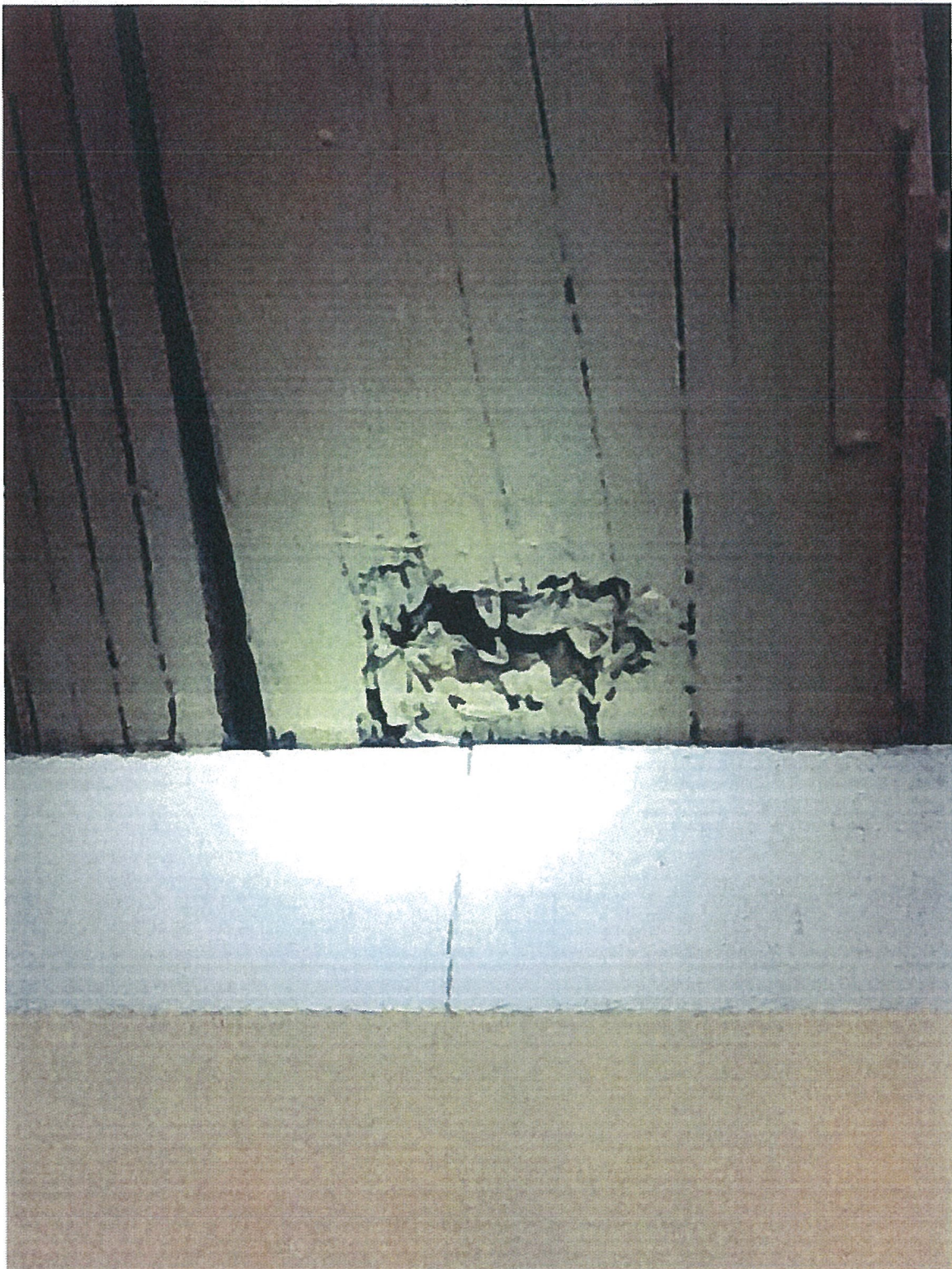
Roof truss evidencing deterioration at load bearing [HCC 5-48(2)(F)]
