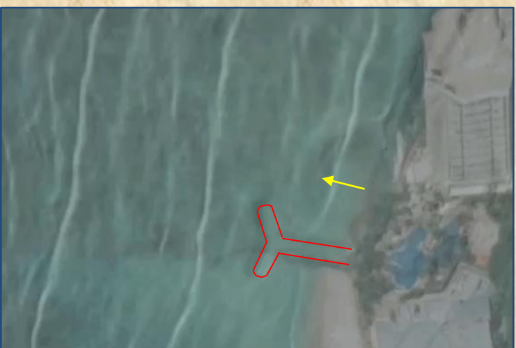
Rock T-head groyne
