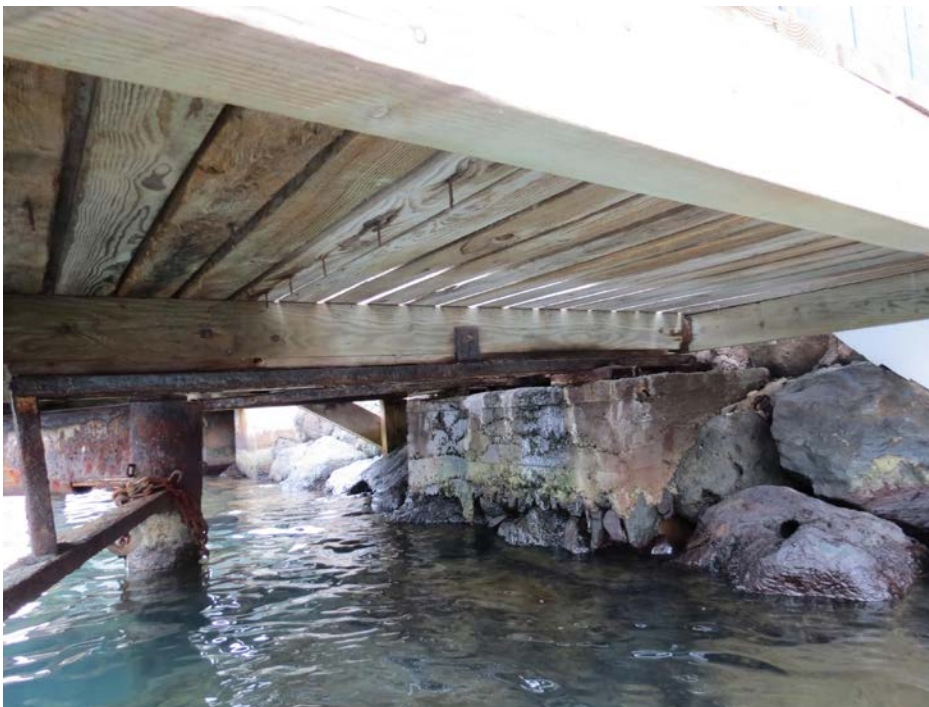
The underside of the platform showing the metal beams and supports.
