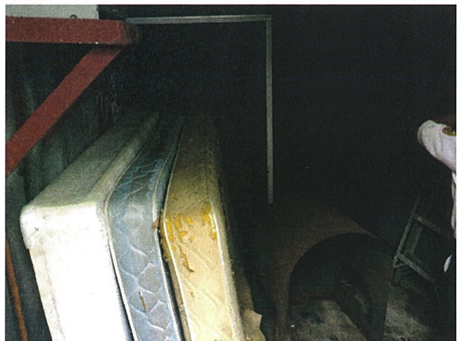
Remove combustibles from main electrical room, such as beds, and other flammables
