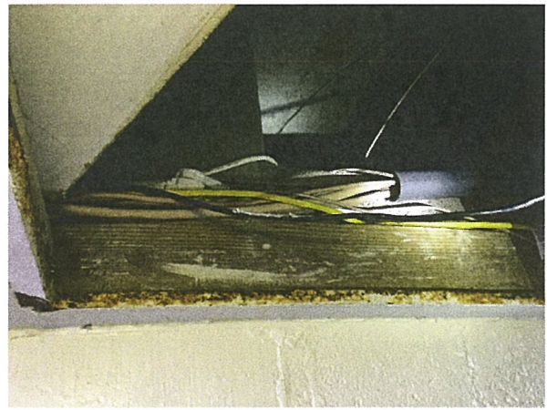
Extension cord use in ceiling not allowed due to increased Fire dangers associated with this practice
