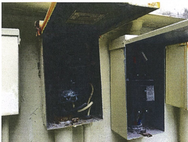
Electrical box has non rated bolts connecting wires
