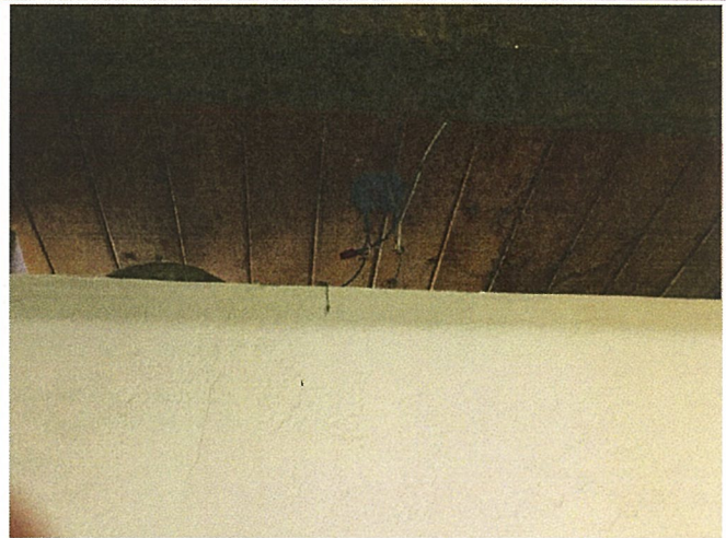
Electrical wiring is exposed and not installed per code
