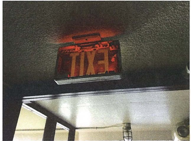
Emergency exit sign needs to be replaced
