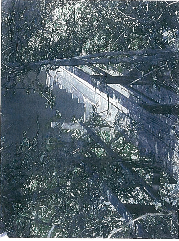
Ukumehame Reservoirs (MA-0140) Perilous Access to Outlet Operator - Missing Hand Rail
