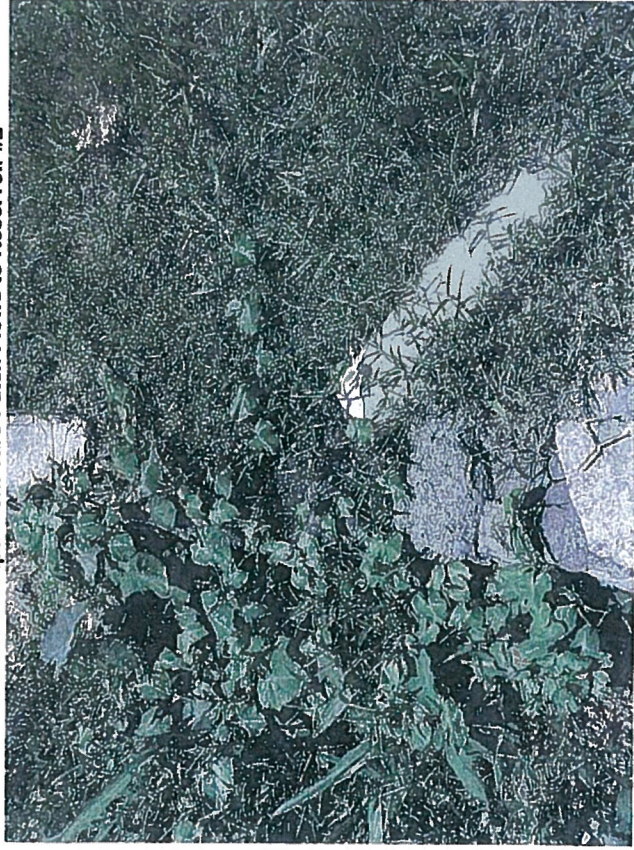
Ukumehame Reservoirs (MA-0140) 5 Inch PVC Pipe From Taro Patch Flows to Reservoir #2
