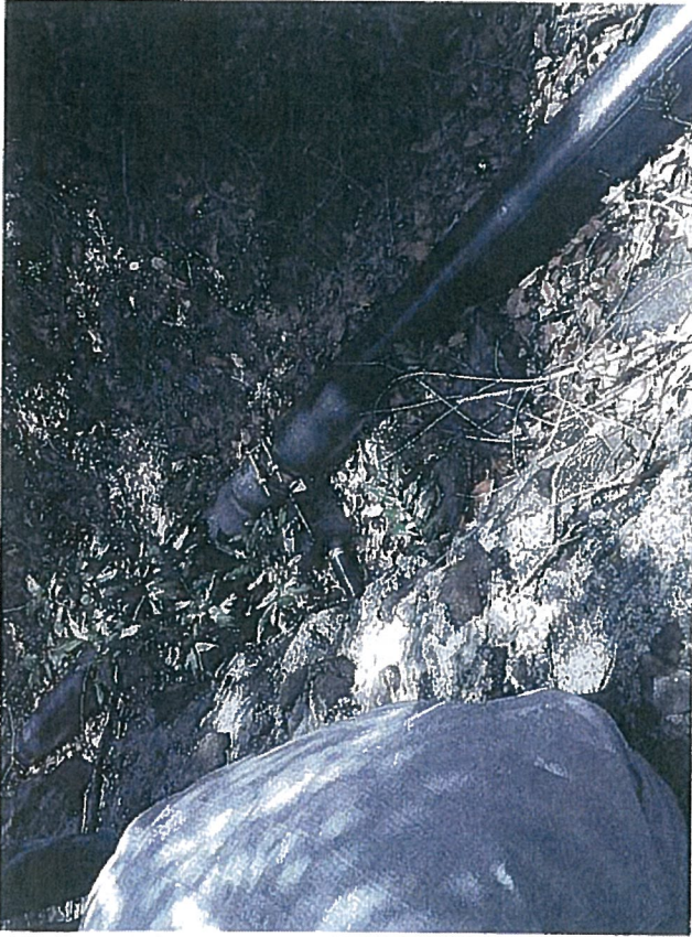
Ukumehame Reservoirs (MA-0140) 8 Inch HDPE Pipeline - 2 Inch HDPE Line Tees Off
