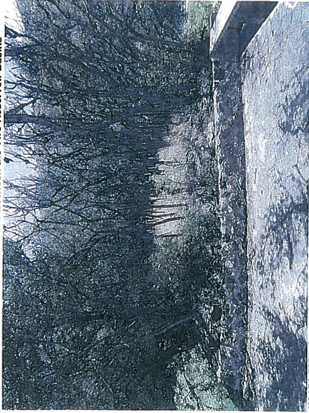
Ukumehame Reservoirs (MA-0140) Hundreds of Trees on the Dike Between the Two Reservoir Basins
