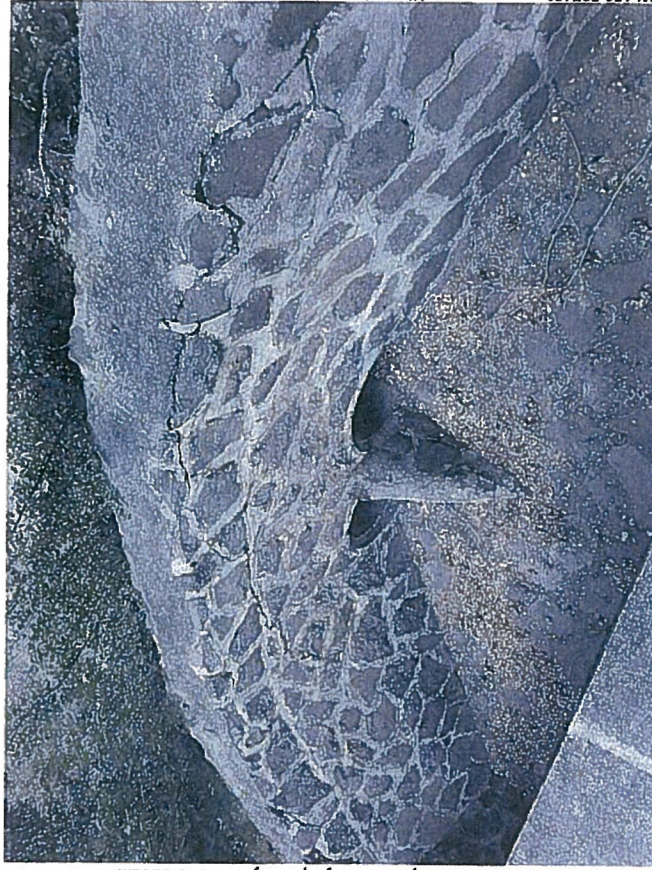
Ukumehame Reservoirs (MA-0140) Twin 24 Inch Pipes Convey Spillway Flows to Stream
