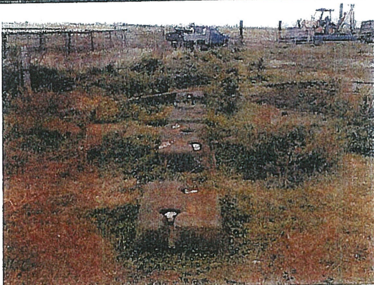
Photograph 1. A view of the fill ports and remote fill ports for Tanks 1 through 4 of the UST facility. 20Apr15.
