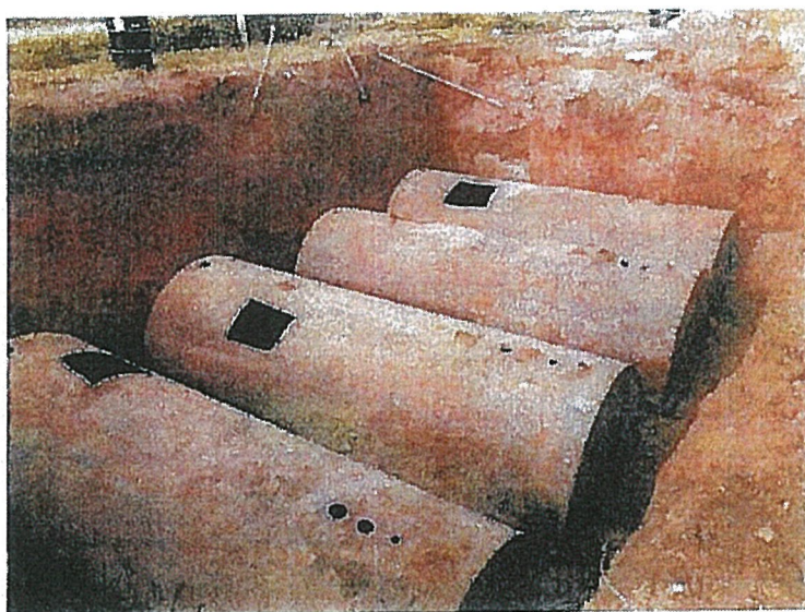
Photograph 3. A view of USTs and closer excavation prior to UST removal. The manway created for UST cleaning is visible. 24Apr15.
