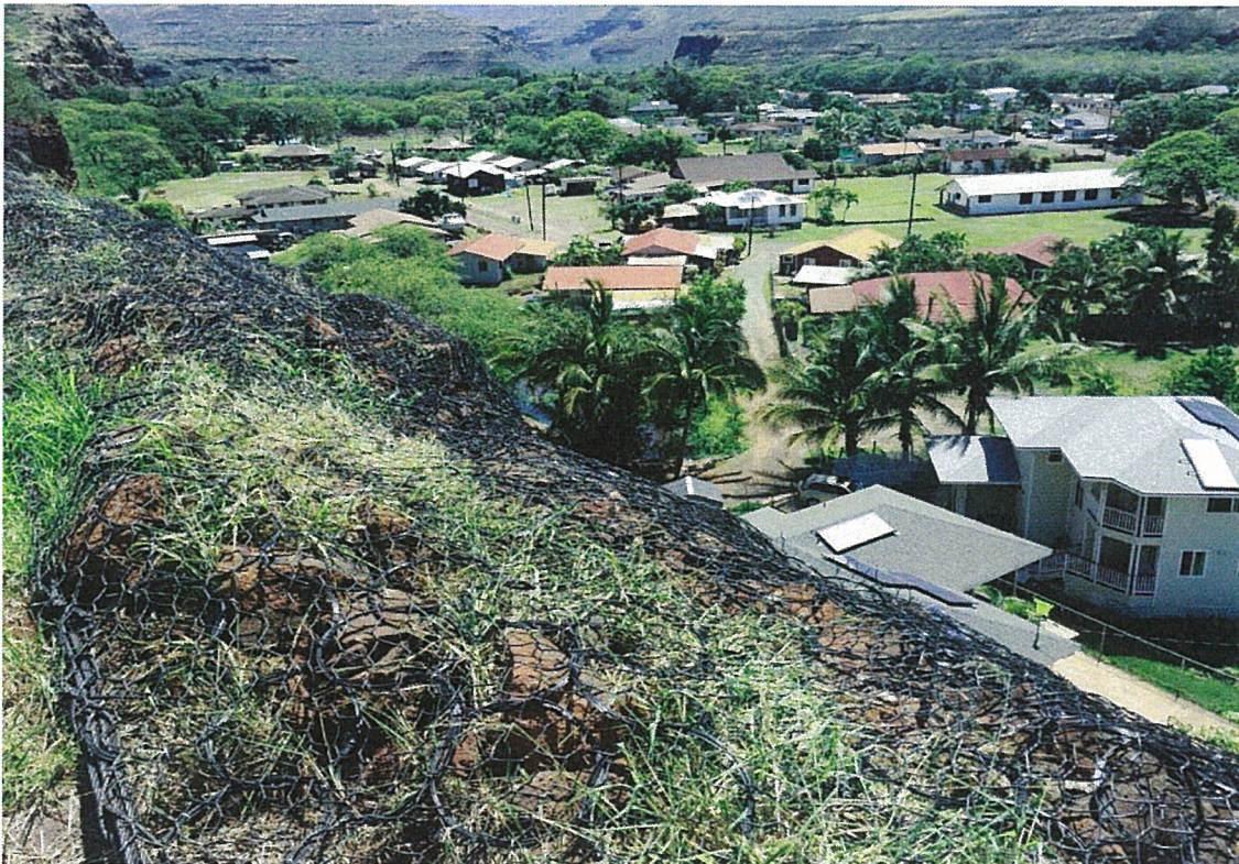
Mesh drape over the cliffs at the top.
