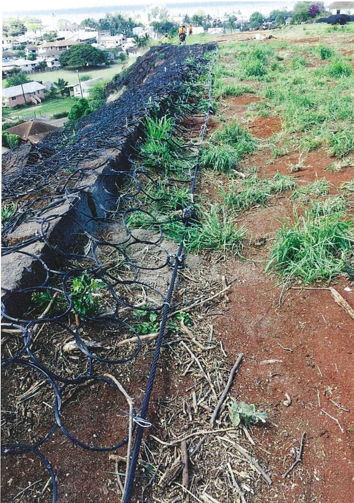
View of draped mesh just over the cliffs.
