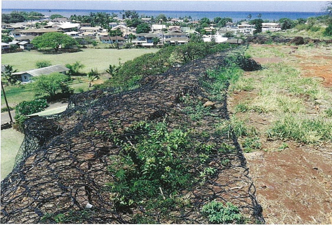
Mesh drape termination at the top of cliffs.
