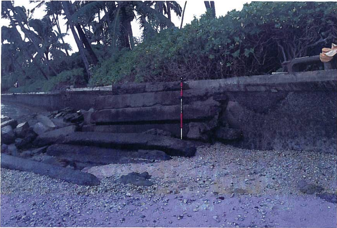
Seawall and culvert outfall structure at the project site.
