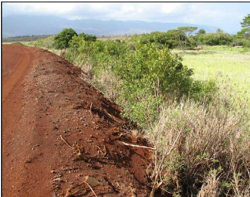
14. View of downstream slope looking left from top of dam near Station 3+50. Note dense woody vegetation on downstream slope.
