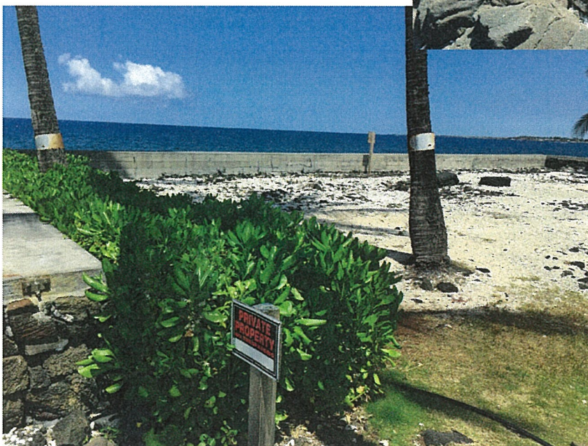
Level yard created by backfill on mauka side of wall
