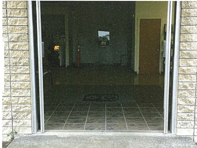
Office entry doorway
