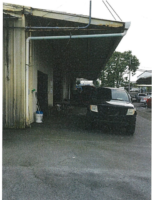
Town side of smaller bldg. – front to back
