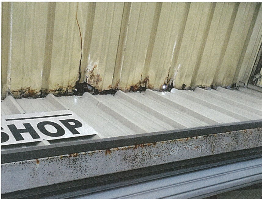
Roof inside smaller bldg. – active leaks
