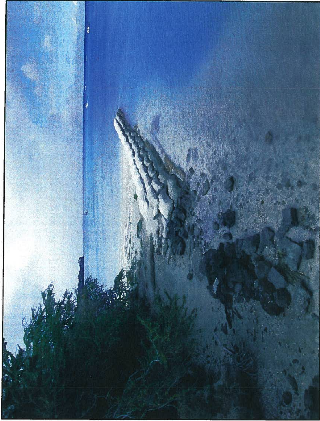
Erosion and flanking as viewed from the Kalanianaʻole Highway Bridge (May 2015)
