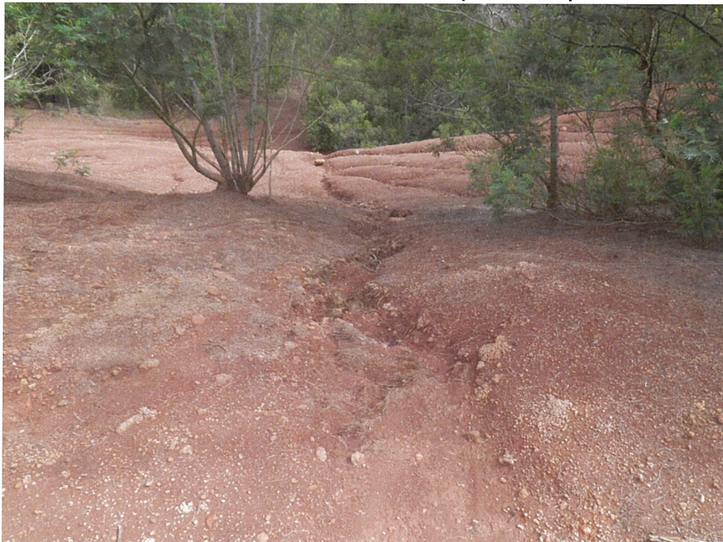
Kitano Reservoir (KA-0004) Erosion Gullies and Trees on the Upstream Slope
