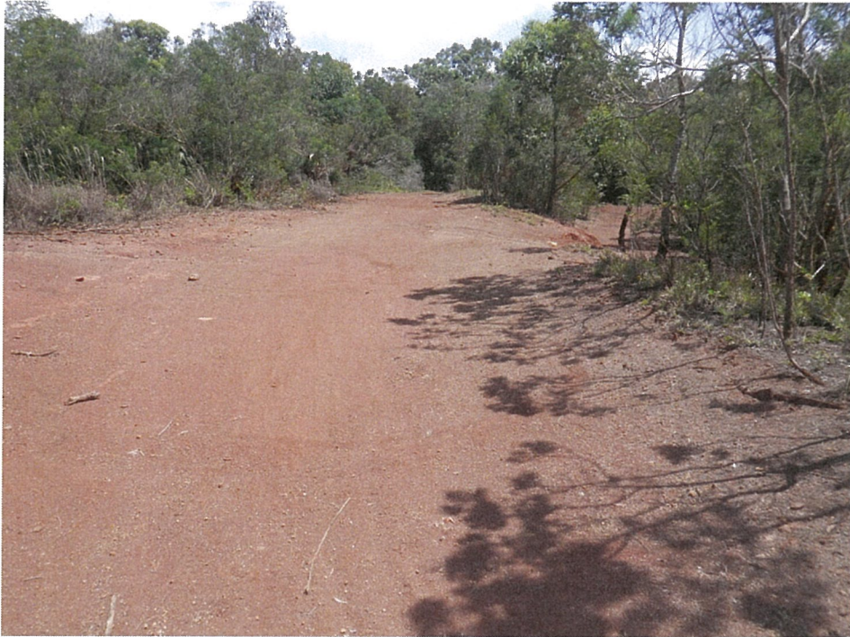
Kitano Reservoir (KA-0004) Right Side of Embankment - Wide Dam Crest
