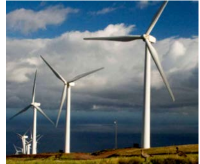
Kaheawa Wind Power project in West Maui above Ma'alaia.
