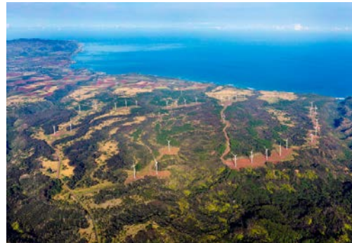
Kawailoa Wind Power, O'ahu
