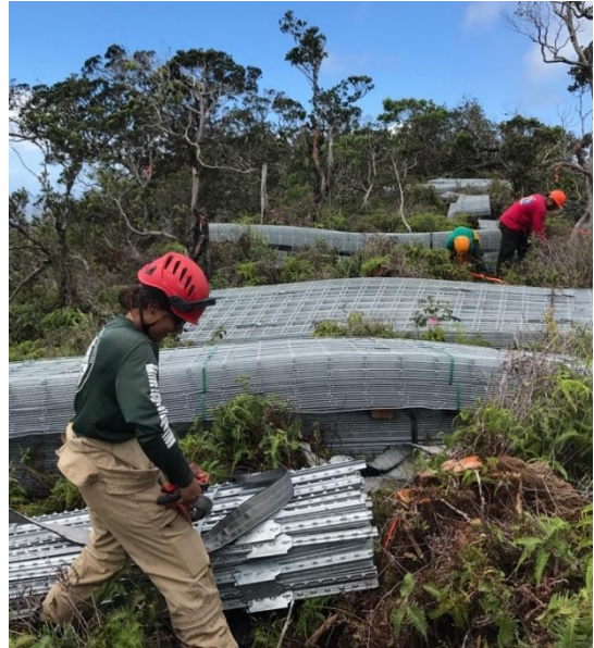
Building fence at Poamoho in the Ko'olau Mountains, O'ahu.
