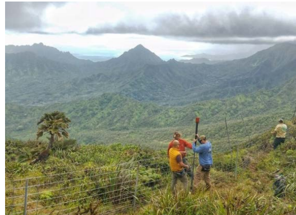
Ko‘olau Mountains Watershed Partnership building fence mauka of Wahiawā, O‘ahu.
