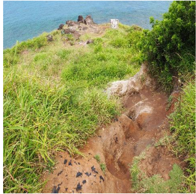
Makeshift Access Trails to Honoloua Bay Showing Scouring
