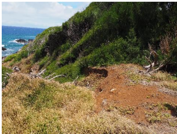
Head Cut and Debris in Flow Way
