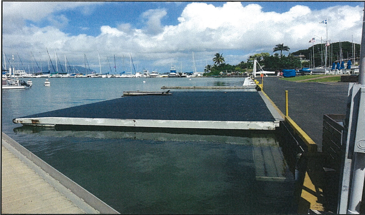
Photo: Floating Metal Pier with Rubber-type Lining
